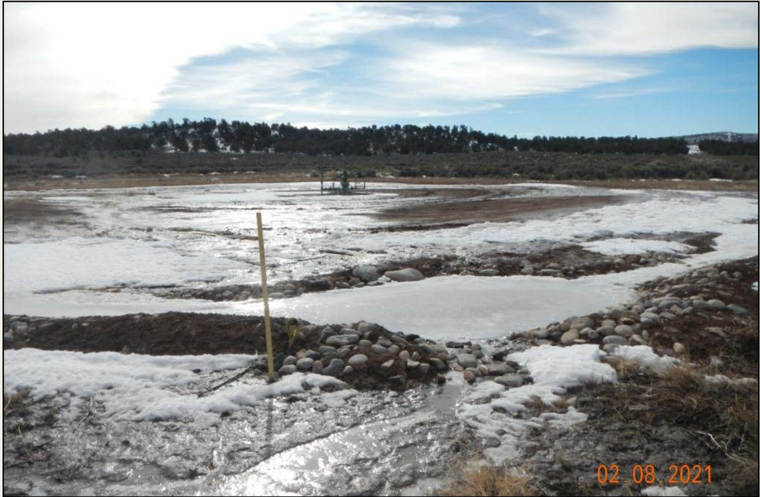
Photo 1. View of the wellhead portion of the project area from the northwestern corner facing center. Silt trap is not adequately sized as it is full and flowing over during a minor runoff event.
