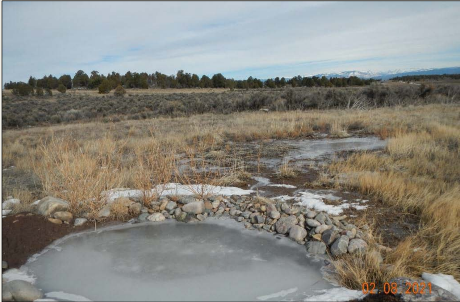
Photo 2. View of silt trap along the northern edge of the project area, is no adequate as it too is overflowing during a minor runoff event. Sediment transport is observed in overflow. Downslope areas need seeding.
