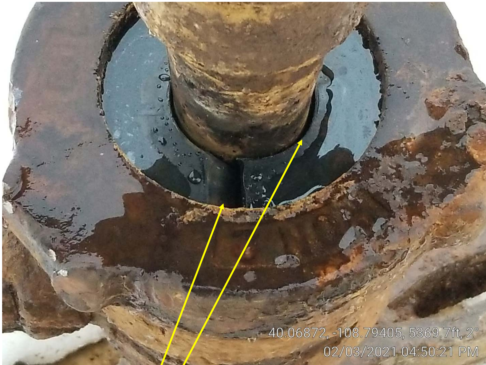
Photo 4. Well with gas leak.
