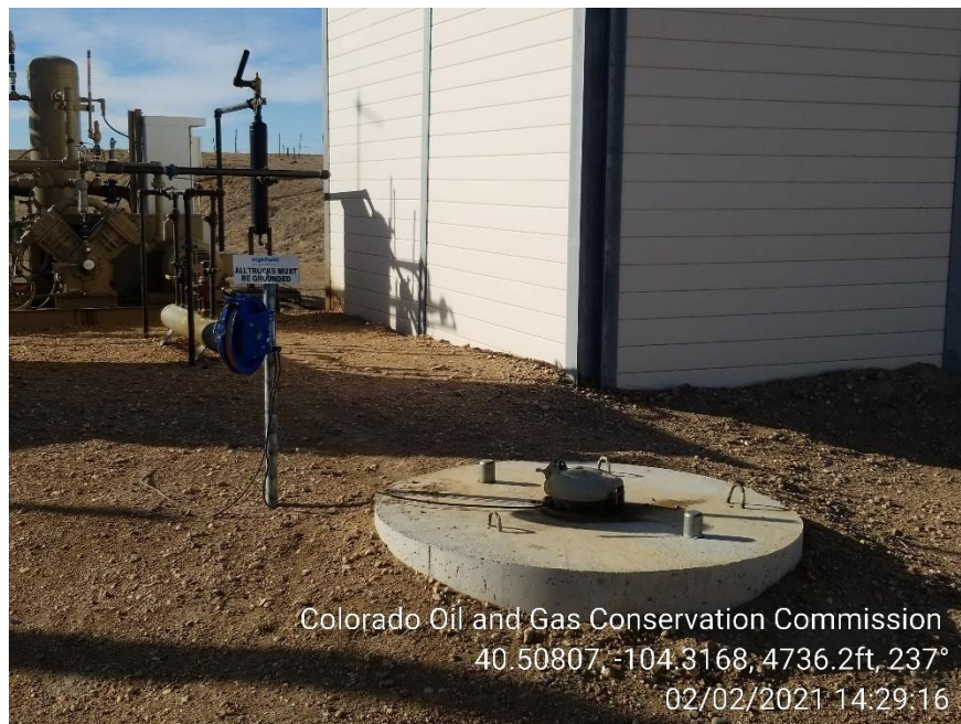
Photo 5 – Concrete Vault missing Labels
