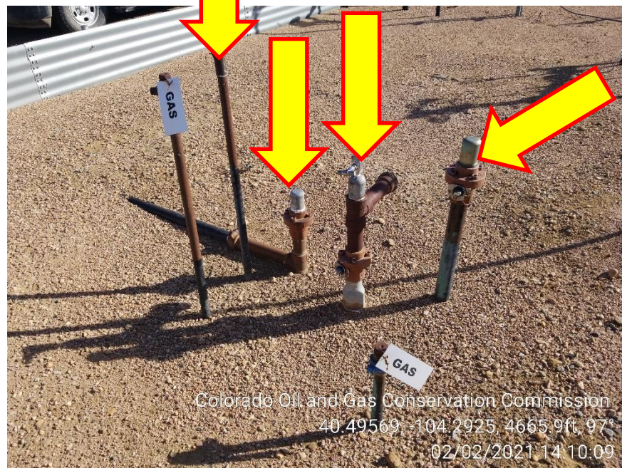
Photo 9 – Unmarked Risers
