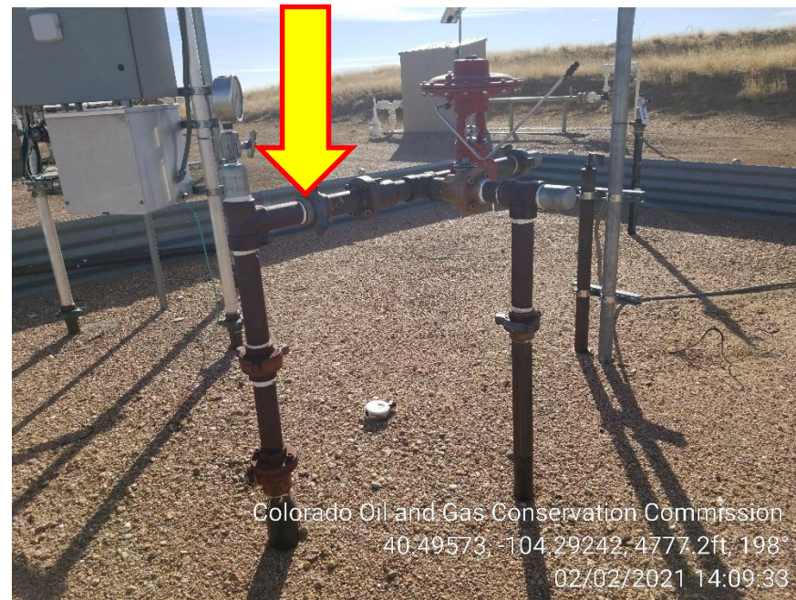
Photo 6 – Unmarked Riser
