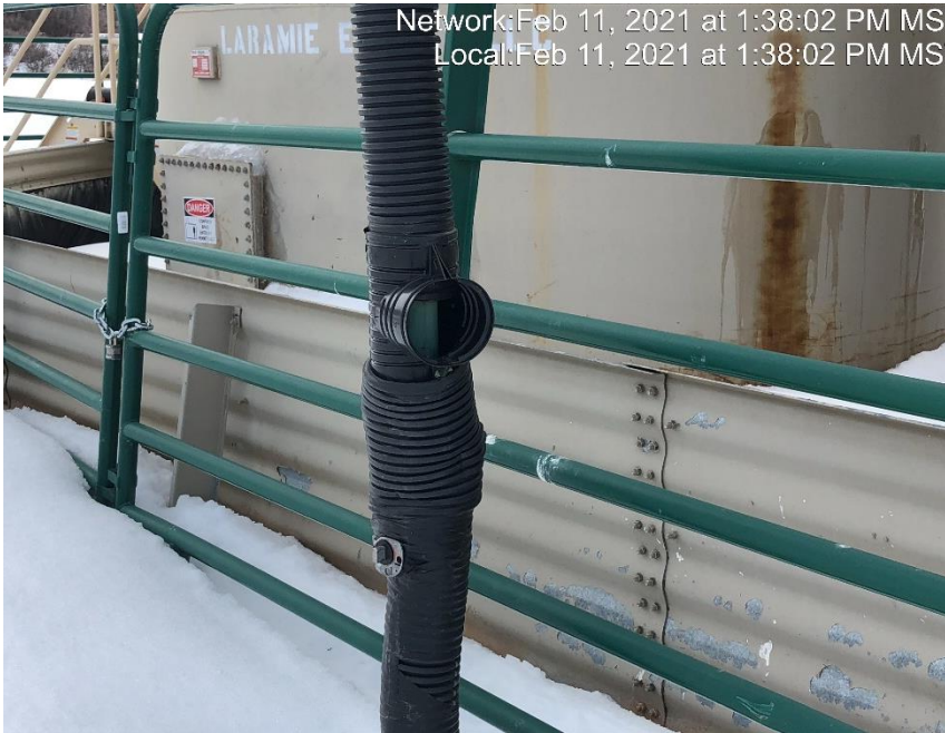
Photo #2890 Dump line heating insulation open ended and not capped.
