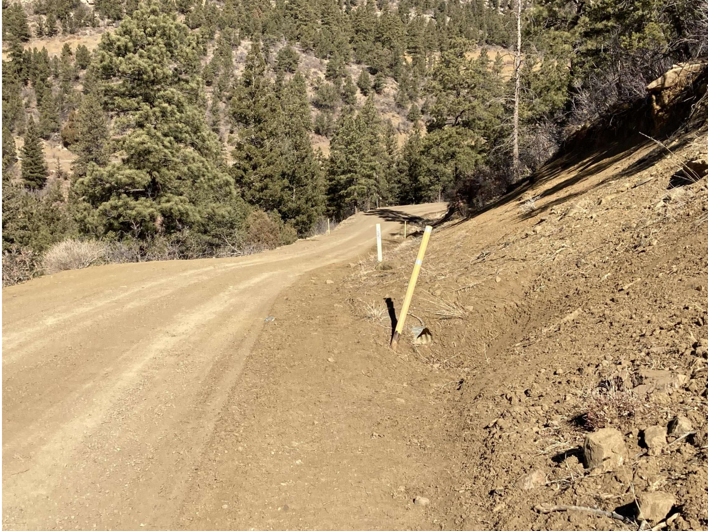
PHOTO 1: THE ROAD SURFACE WAS REGRADED TO CREATE SHEET FLOW AND ELIMINATE THE TIRE RUTS/ SURFACE EROSION.
