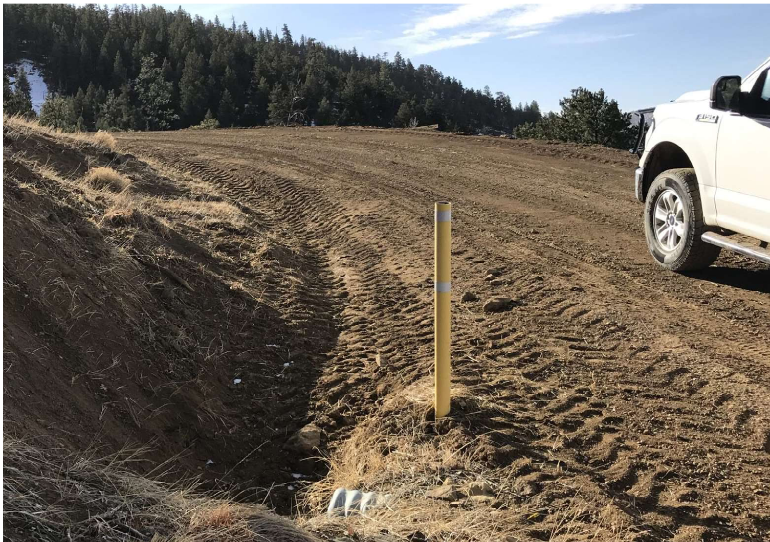
PHOTO 2: THE BAR DITCH WAS DOMINATED TO RECEIVE STORMWATER RUN OFF FROM THE ACCESS ROAD.
