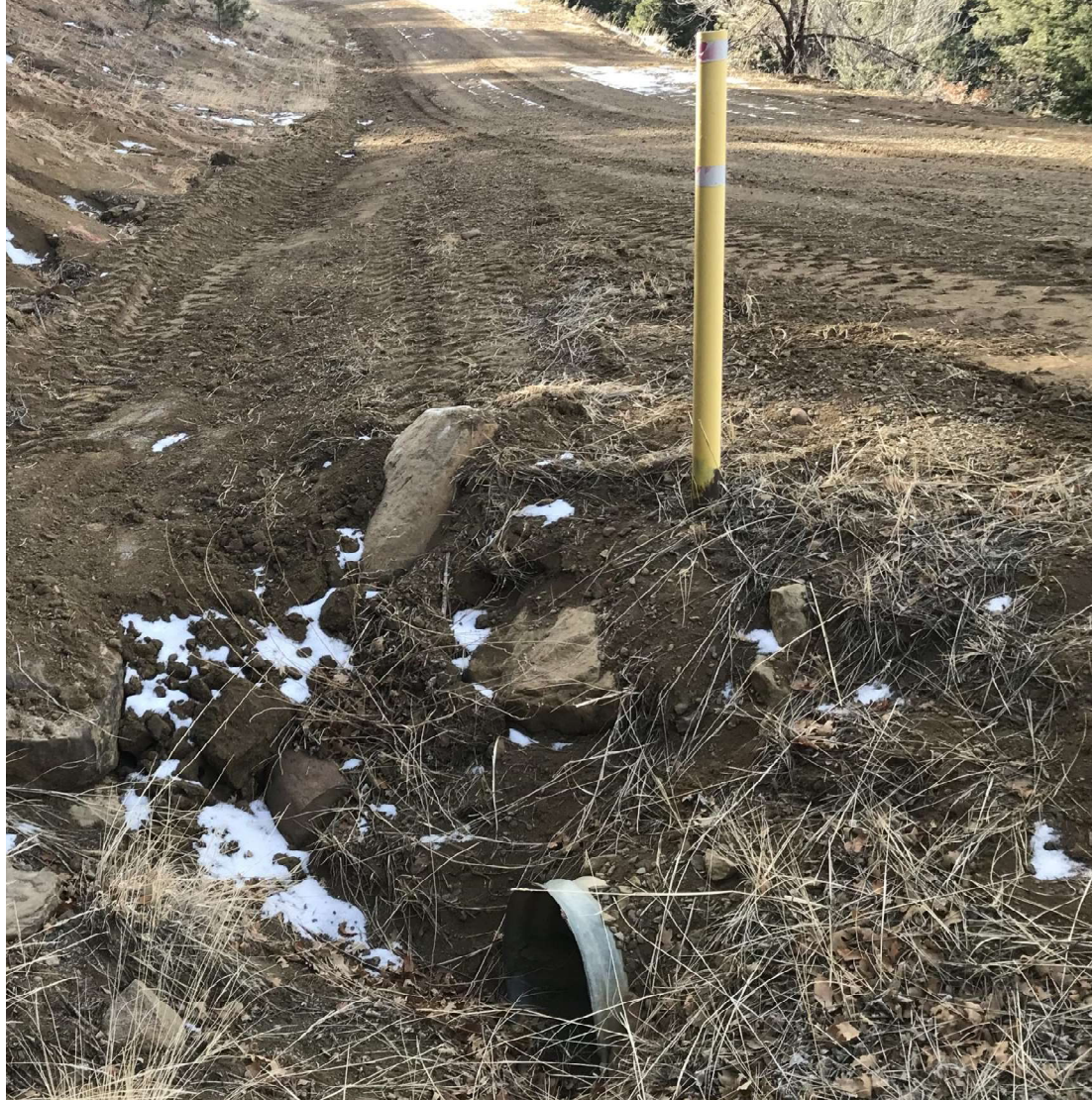
PHOTO 3: THE SEDIMENT ACCUMULATION WAS REMOVED FROM THE CULVERT INLET
