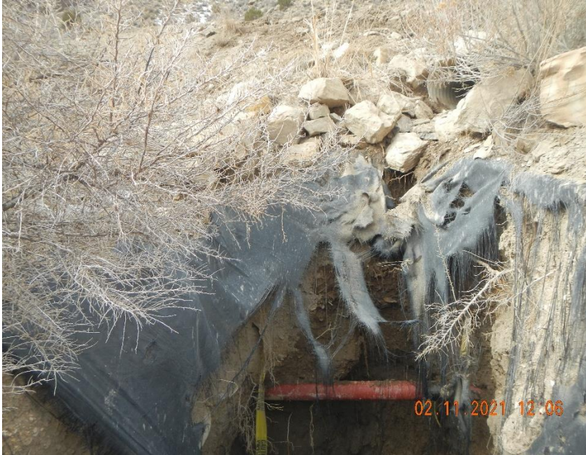
N39.55348 W-108.11985 Erosion damage from culvert outlet.
