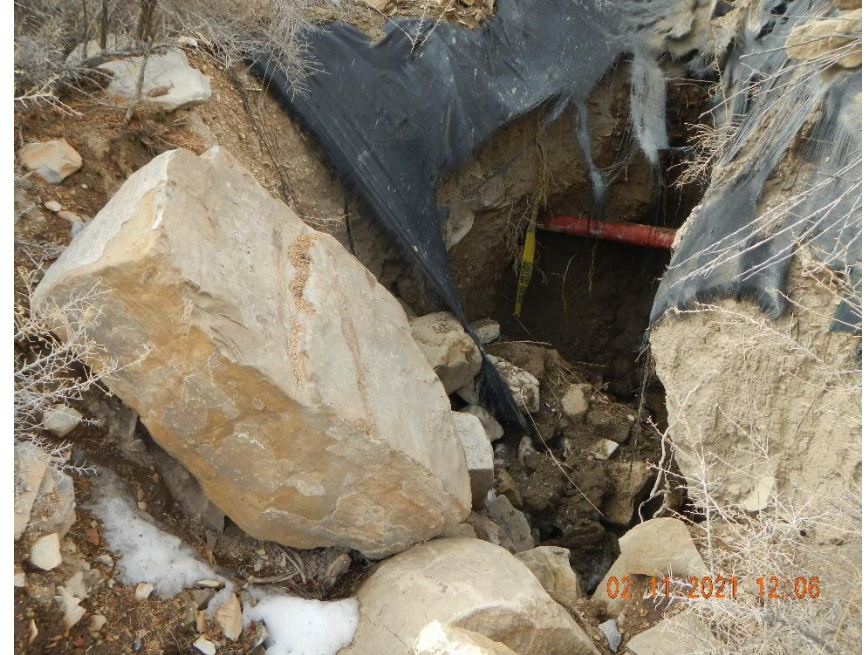
Erosion has exposed pipe line.
