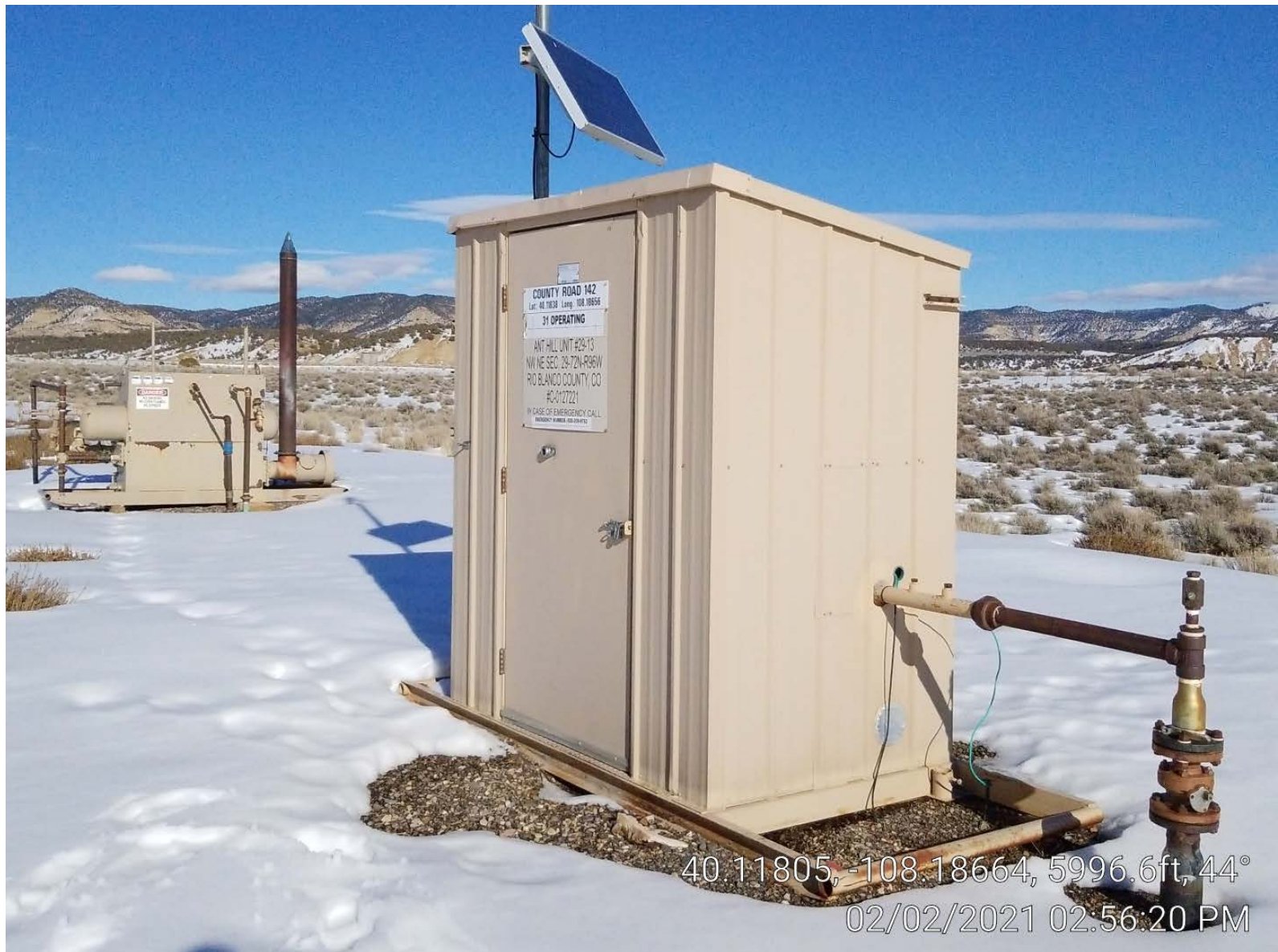
Photo 4. Meter building & separator.
