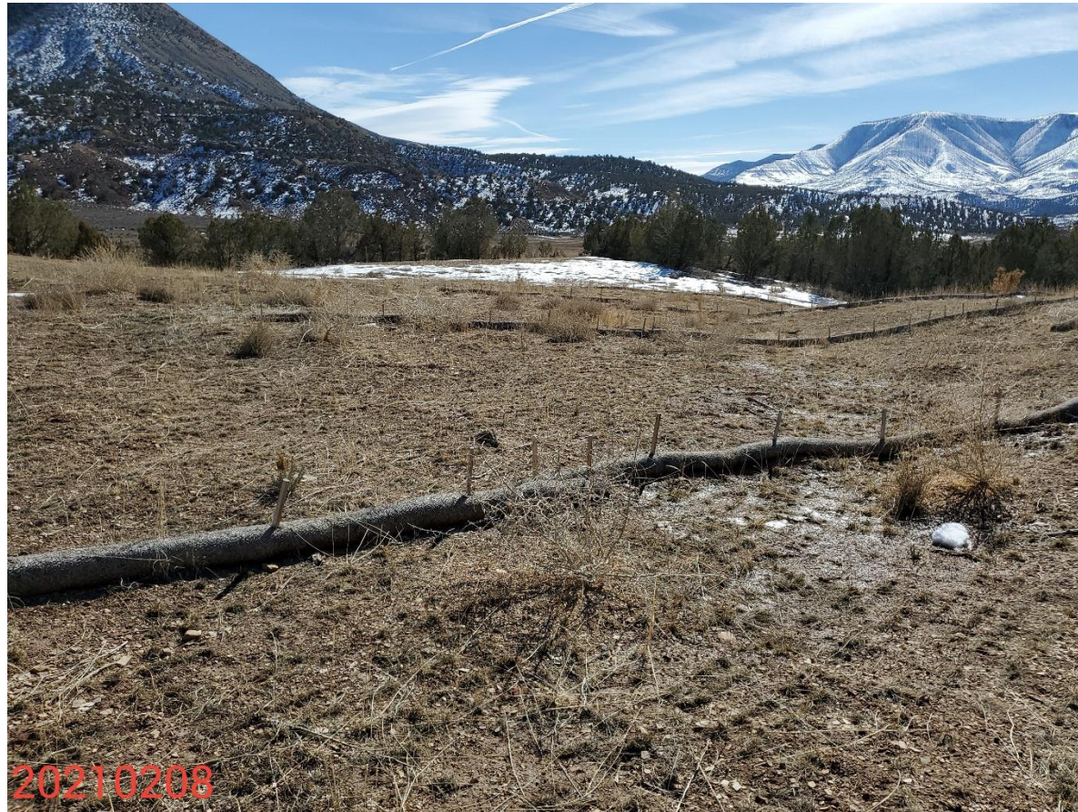
Photo 5: Photo shows straw wattle BMP on the Location. Photo shows wattle BMPs on the Location remain improperly installed / not installed in accordance with good engineering practices.
