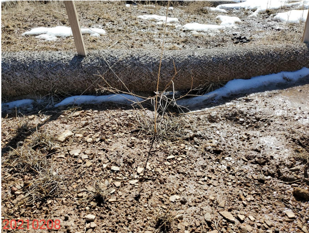
Photo 6: Photo shows straw wattle BMP on the Location. Photo shows wattle BMPs on the Location remain improperly installed / not installed in accordance with good engineering practices; Stormwater cutting beneath BMP. BMPs to stabilize the soils have not been installed and remain missing, or insufficient/inadequate.
