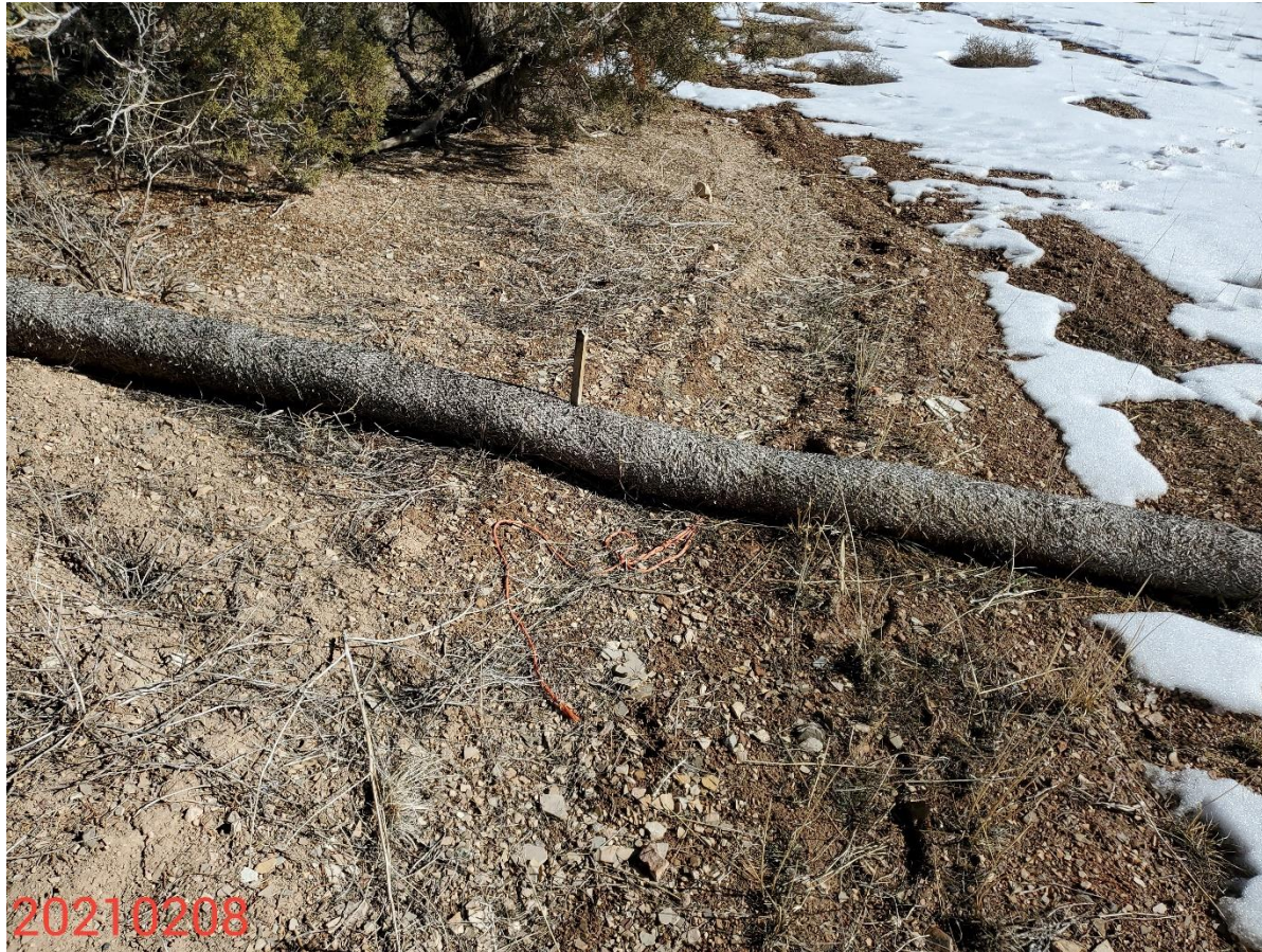
Photo 3: Continued from photo 1. Photo shows wattle BMPs on the Location remain improperly installed / not installed in accordance with good engineering practices. BMPs to stabilize the soils have not been installed and remain missing, or insufficient/inadequate.
