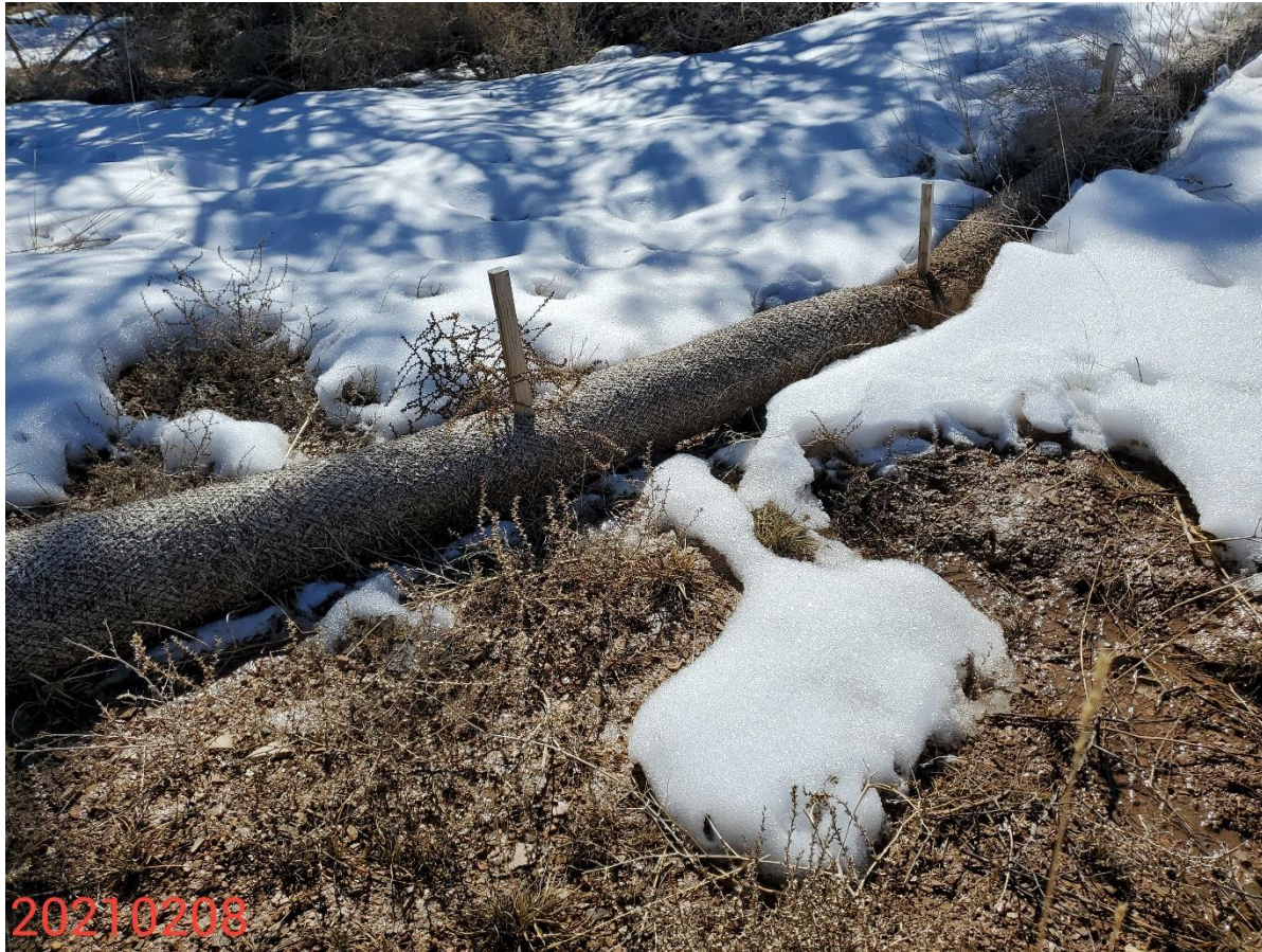
Photo 7: Photo shows straw wattle BMP on the Location. Photo shows wattle BMPs on the Location remain improperly installed / not installed in accordance with good engineering practices.
