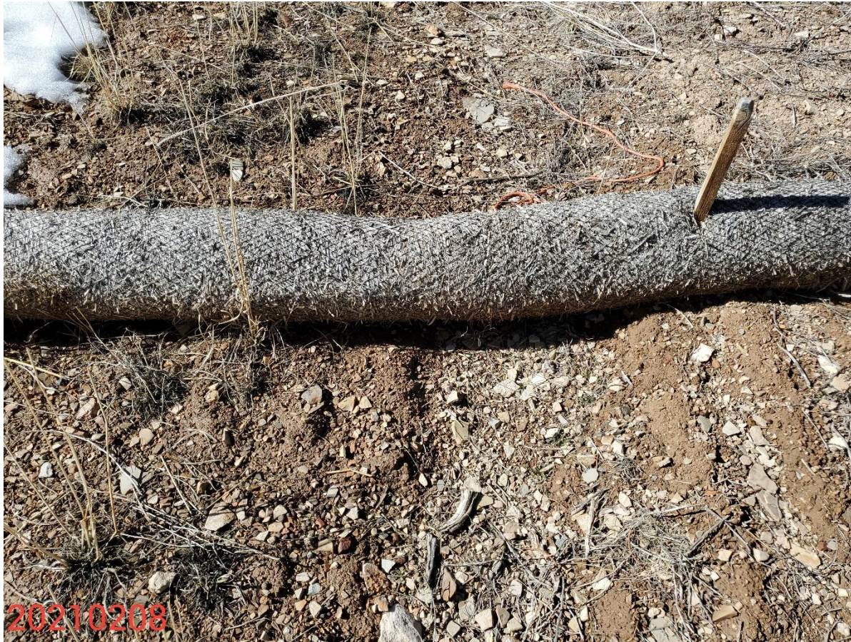
Photo 2: Continued from photo 1. Photo shows wattle BMPs on the Location remain improperly installed / not installed in accordance with good engineering practices. BMPs to stabilize the soils have not been installed and remain missing, or insufficient/inadequate.
