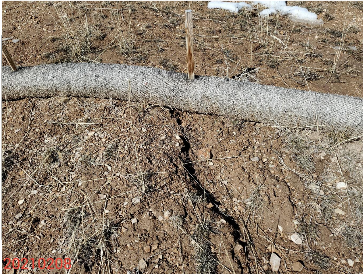
Photo 8: Photo shows straw wattle BMP on the Location. Photo shows wattle BMPs on the Location remain improperly installed / not installed in accordance with good engineering practices. BMPs to stabilize the soils have not been installed and remain missing, or insufficient/inadequate.
