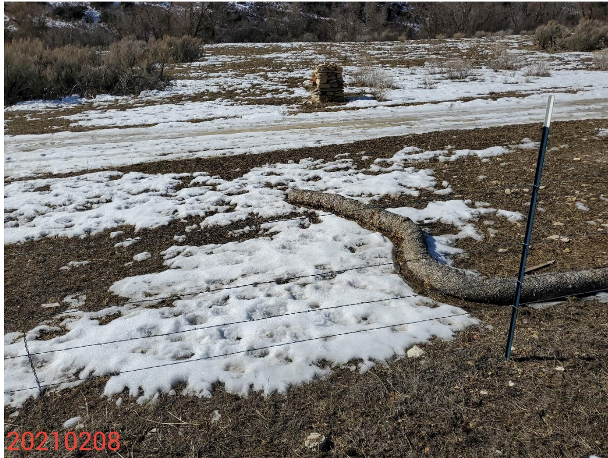
Photo 5: Photo shows straw wattle BMP along southwestern perimeter of the Location is in disrepair. Additionally, wattle BMPs do not appear to have been installed in accordance with good engineering practices.
