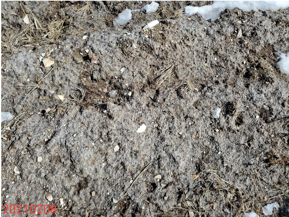
Photo 6: Photo shows hydro mulch has been applied to the soil surface of the reclamation area.
