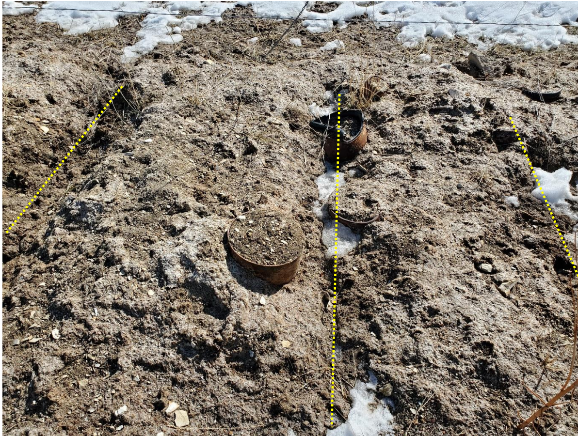
Photo 7: Photo taken from the west end of the Location. Photo shows pipe debris remaining. Photo also shows example of ripping marks on the Location. Rule 1004.a requires cross-ripping to a minimum depth of 18 inches; Location appears to have only been ripped in one direction (yellow lines); No indication that areas were cross ripped.
