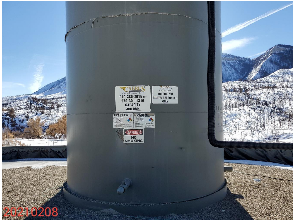
Photo 5: Photo of 400 bbl condensate tank w/ emergency contact numbers.
