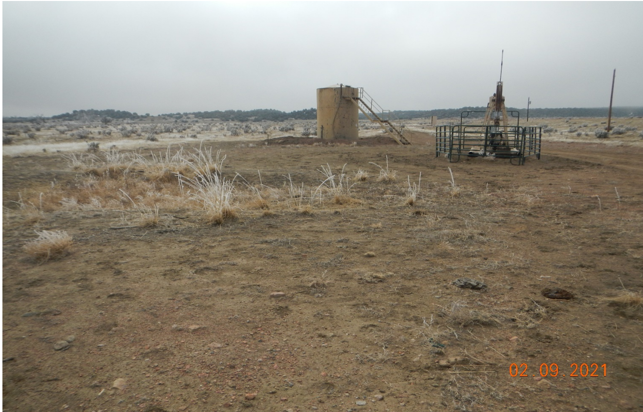
Photo 2. Facing south toward the location. Unused equipment has been removed.
