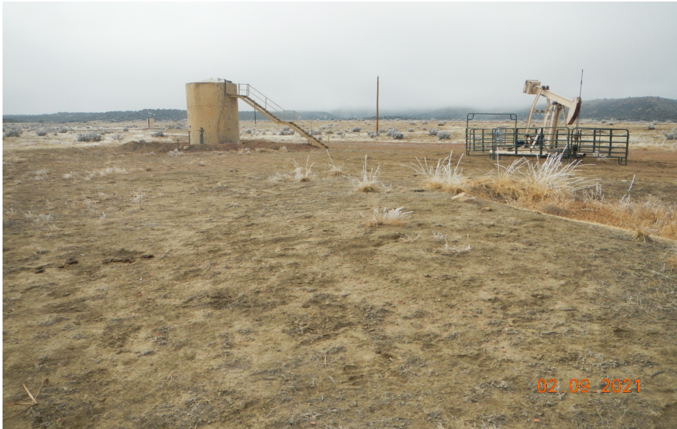
Photo 3. Unused areas around the well need to be reclaimed. The vegetation has not established in the interim reclamation area surrounding the equipment.
