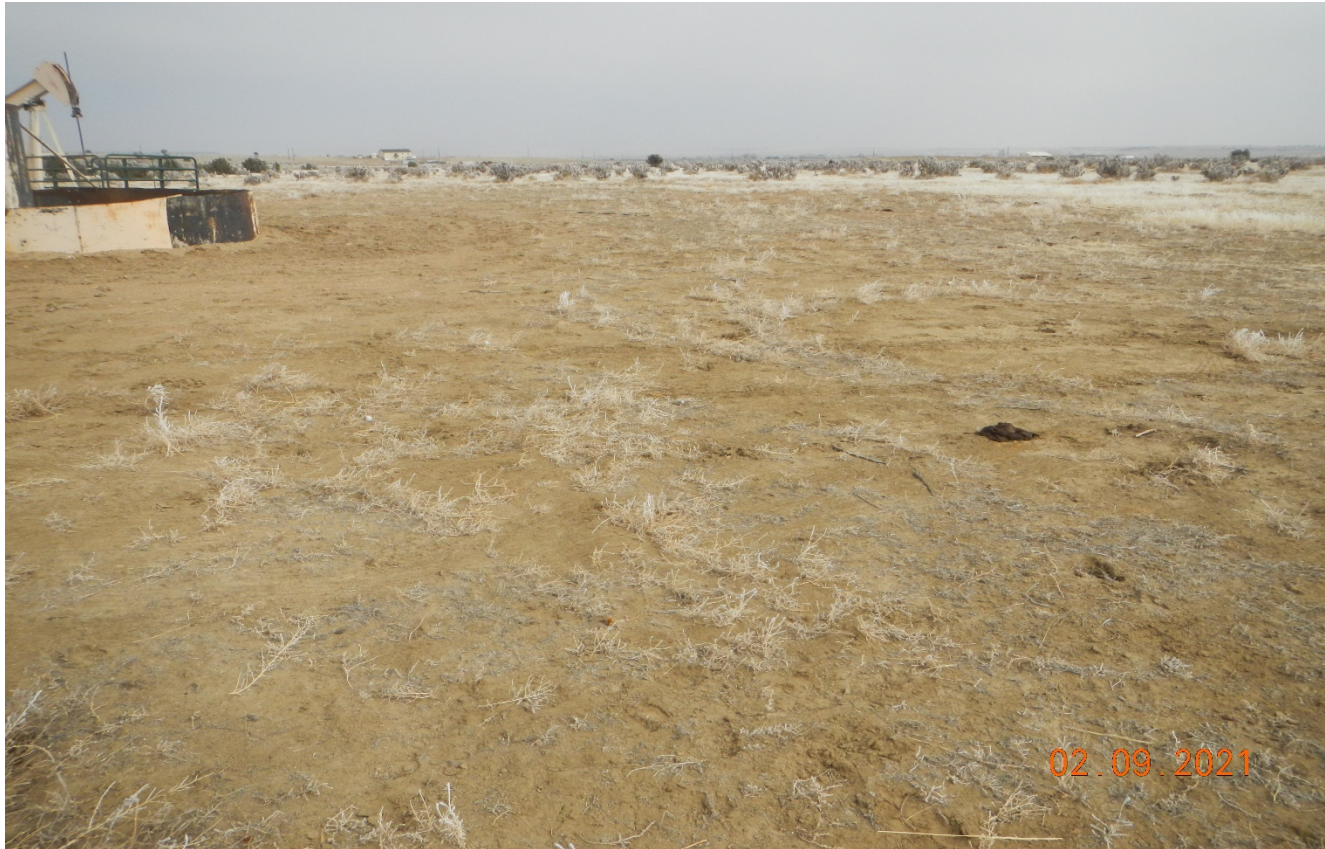
Photo 3. Unused areas around the well need to be reclaimed. There is a lack of vegetation interim reclamation area.
