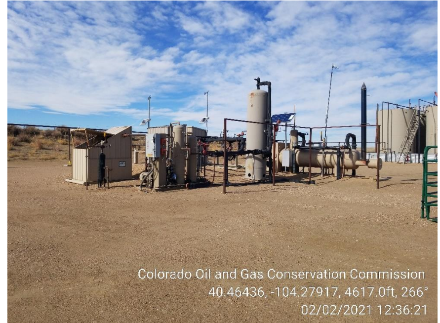
Photo 6 – Separator and VRU
