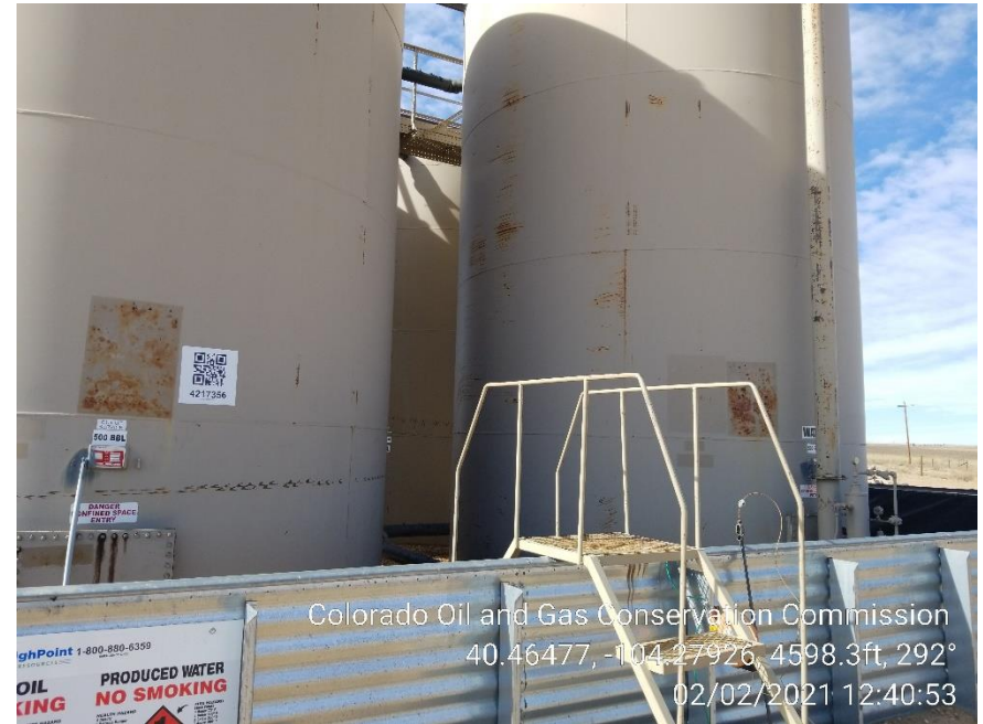
Photo 2 – Tank Battery
