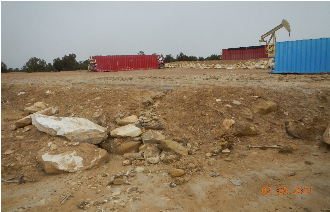
Photo 3. Facing north at the location. There is erosion occurring of the disturbed pad site which is filling in the perimeter wattles. Previous corrective action has not been performed.
