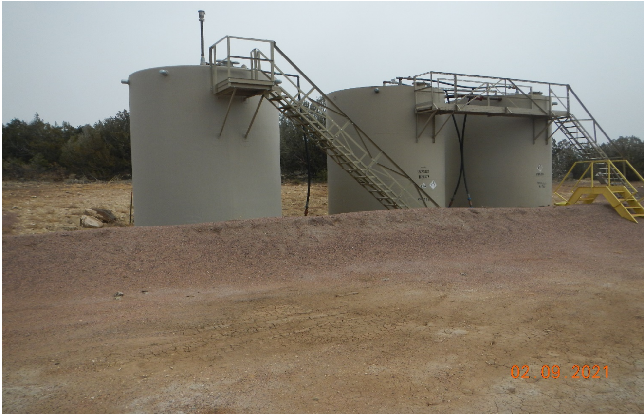
Photo 6. The tanks at north side of the location are not properly labeled.
