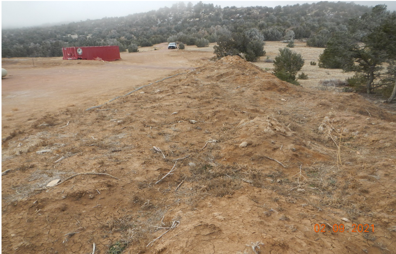
Photo 9. Facing toward the topsoil pile. The topsoil piles are not stabilized and protected. Topsoil piles have not been replaced for interim reclamation.
