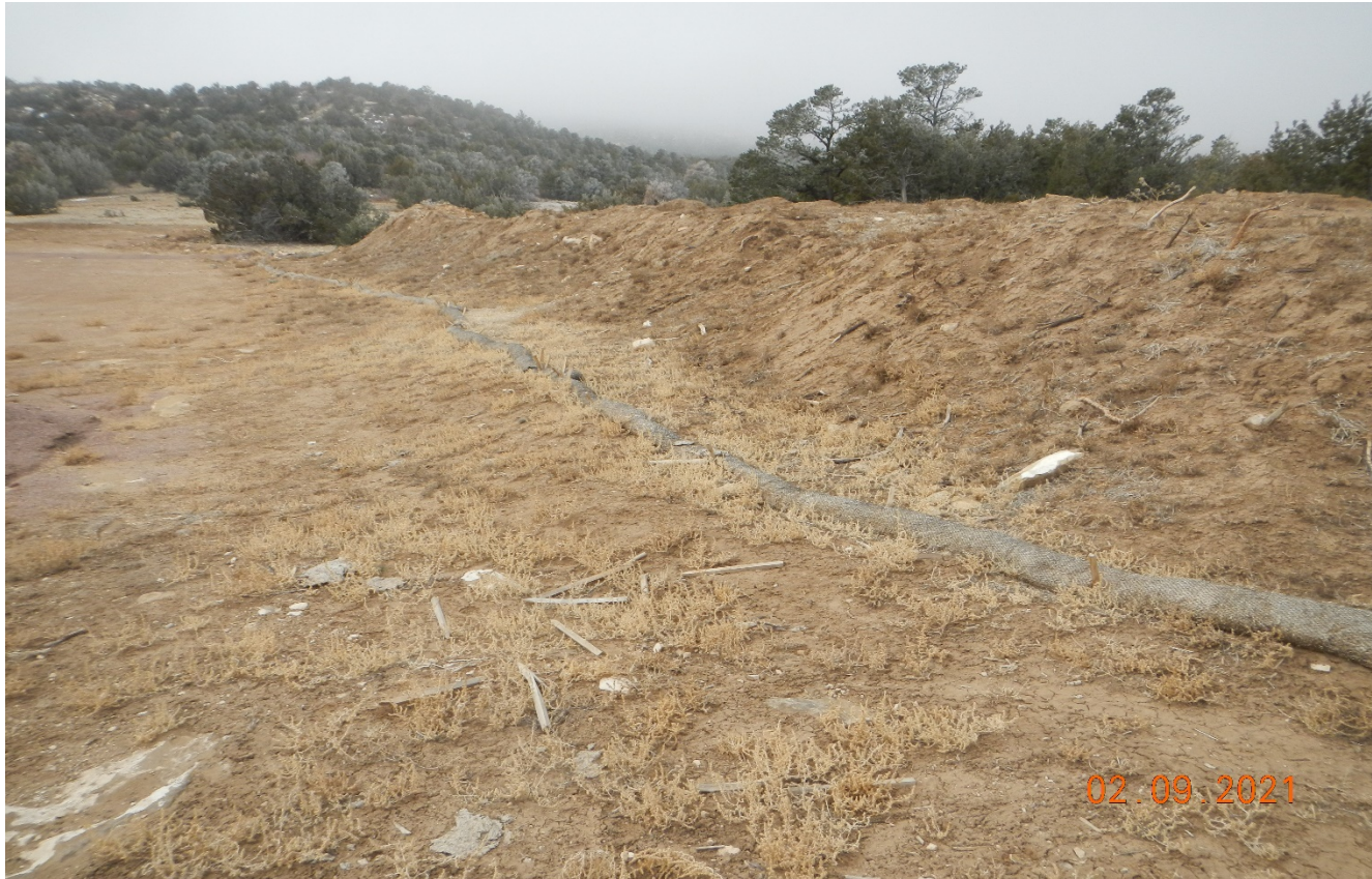
Photo 8. Facing southwest toward the topsoil pile which are not maintained and protected from degradation and weed infestation. Previous corrective action has not been performed.
