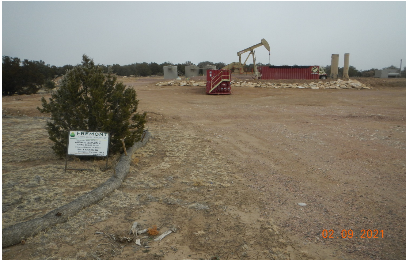
Photo 1. Facing northeast toward the location. Unused equipment has not been removed and interim reclamation has not been performed.
