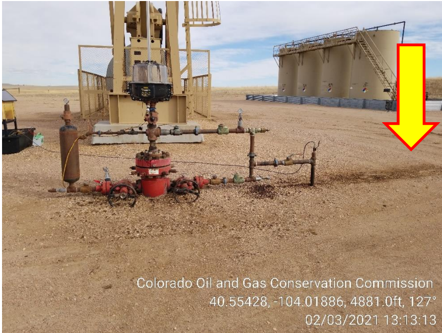
Photo 7 – Wellhead – Stained Soil
