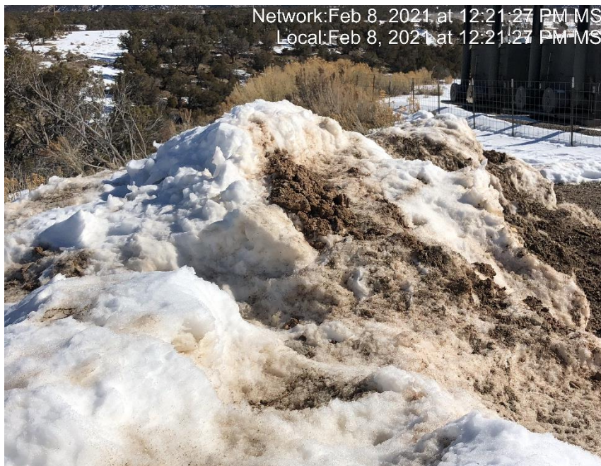
Photo #2841 Back side of berm. Sediment has been push over berm.
