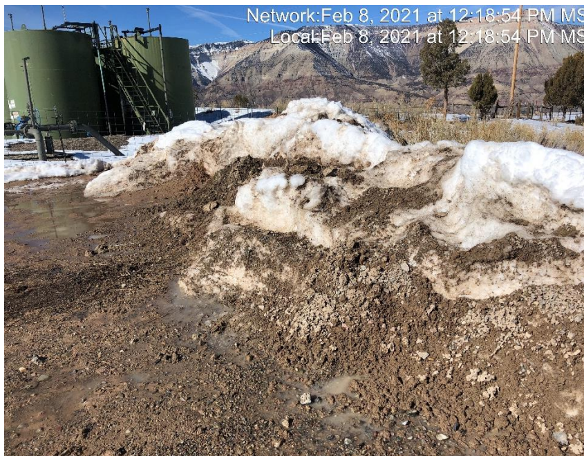
Photo #2839 Front of berm. Sediment has been transported off of location due to snow plowing.
