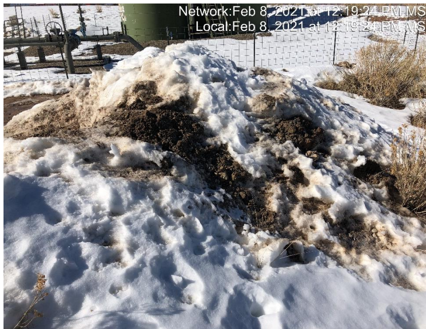
Photo #2840 Back side of berm Sediment has been push over berm.
