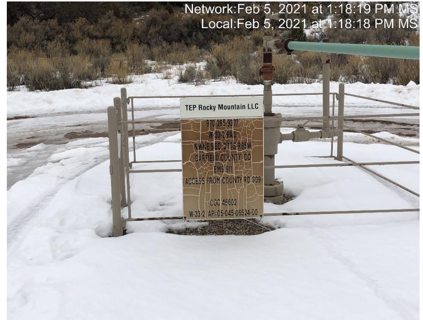
Photo #2832 Wellhead sign weathered and not legible.
