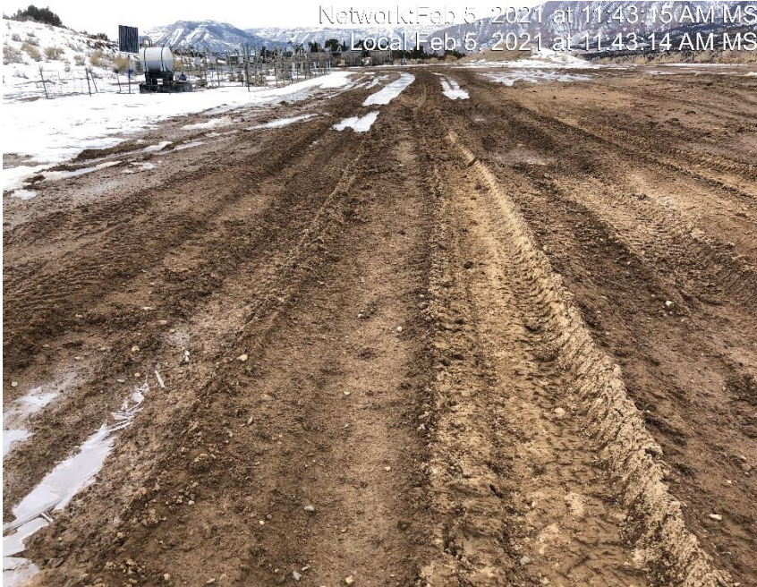
Photo #2822 Rutting present on location due to lack of stabilization.
