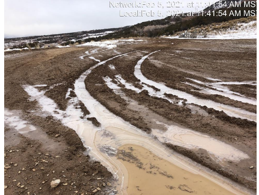
Photo #2821 Rutting present on location due to lack of stabilization.
