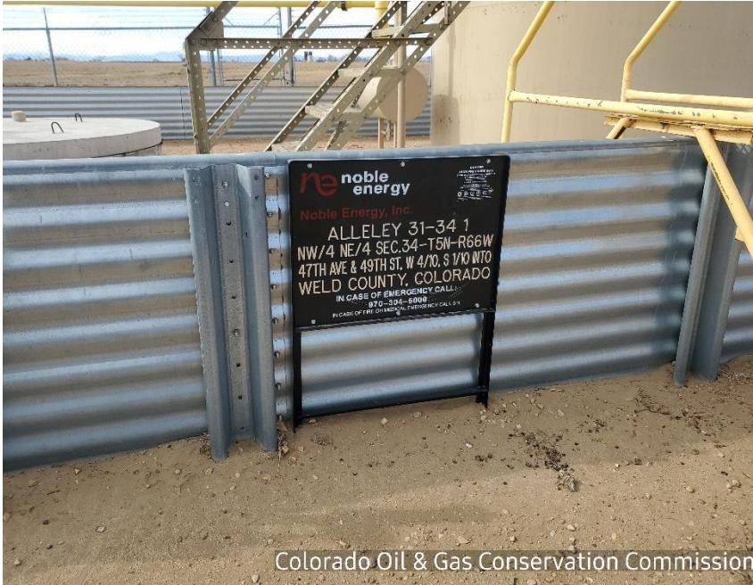
Photo 1: Tank Battery Sign
