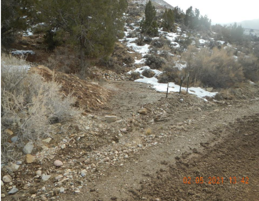
Drainage merging with road ditch is full of sediment.
