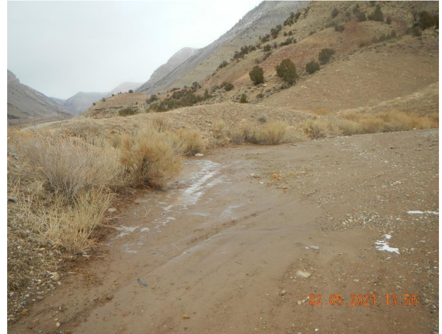
Sediment build up in ditch
