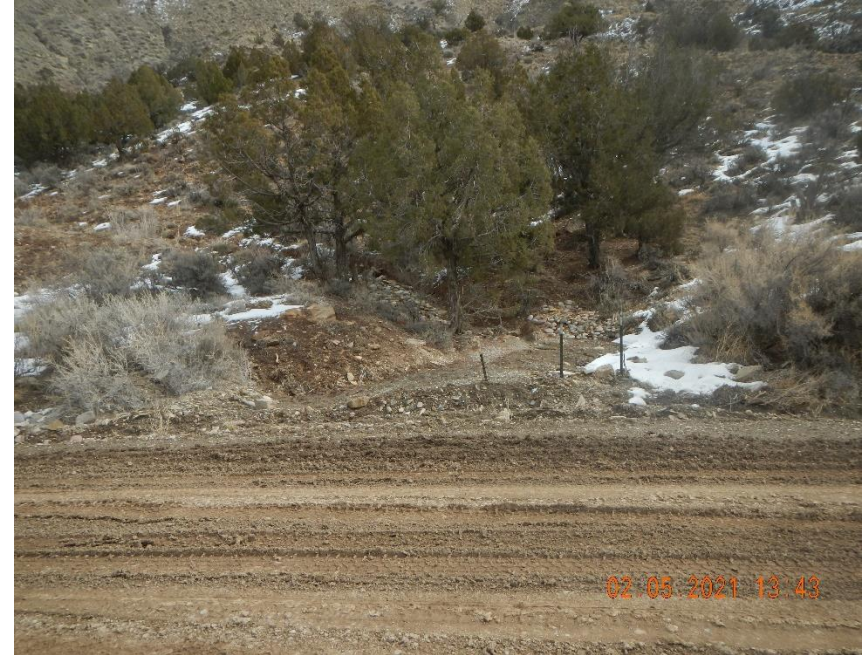
Drainage merging with road ditch is full of sediment.
