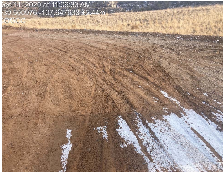
Previous inspection photo of lack of stabilization
