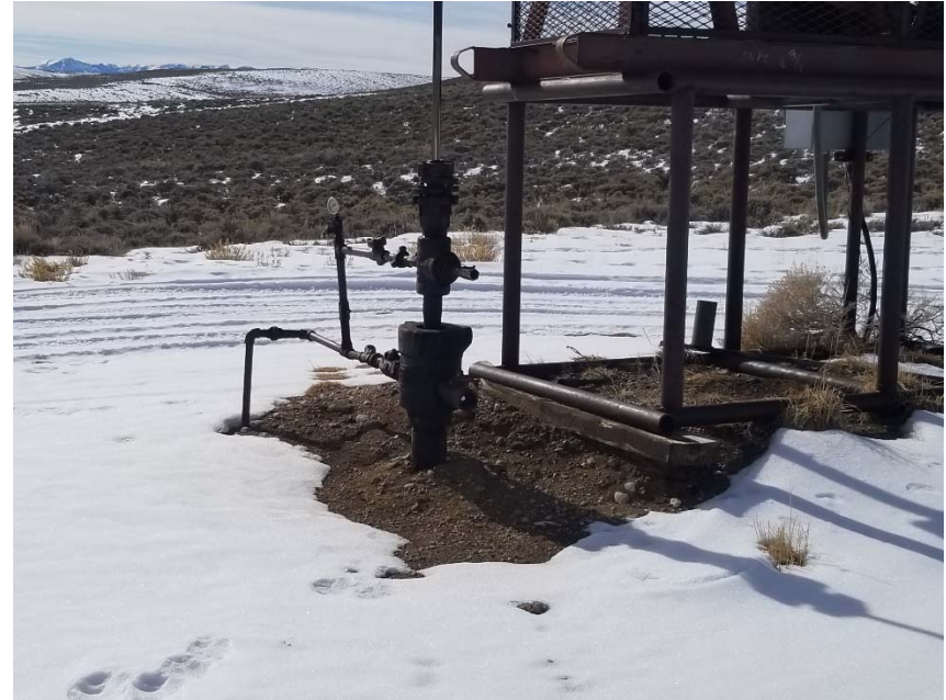
Photo 2. No bradenhead access apparent.
