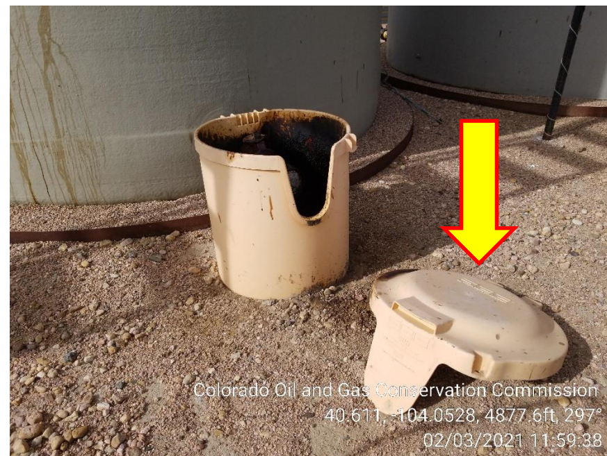
Photo 16 – Loadline Bucket at Produced Water Tank – Oily Waste and Lid Missing. Stained Soil
