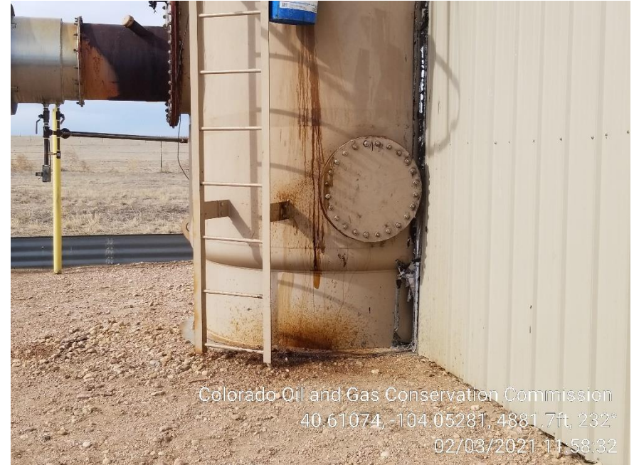
Photo 4 – Heater Treater, Stained Soil STILL REMAINS for previous Inspection
