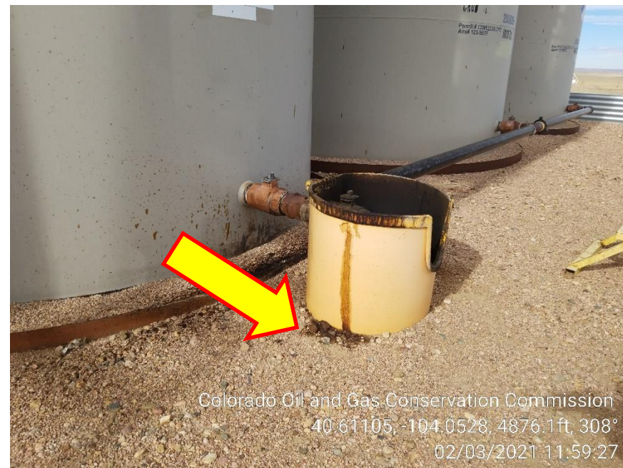
Photo 14 – Loadline Bucket at South Crude Oil Tank – Oily Waste and Lid Missing. Stained Soil
