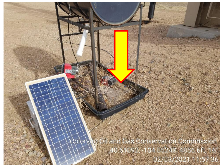
Photo 8 – Debris in Containment. Wildlife Netting is missing
