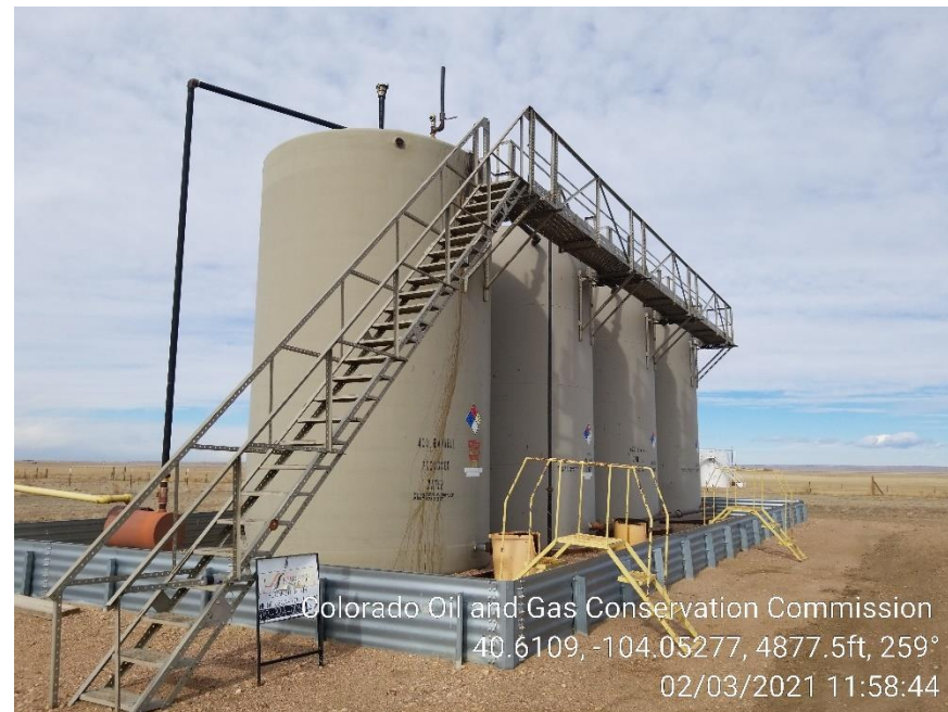
Photo 2 – Tank Battery
