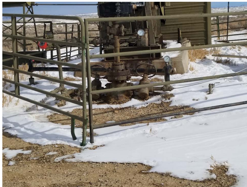
Photo 2. No bradenhead access apparent.
