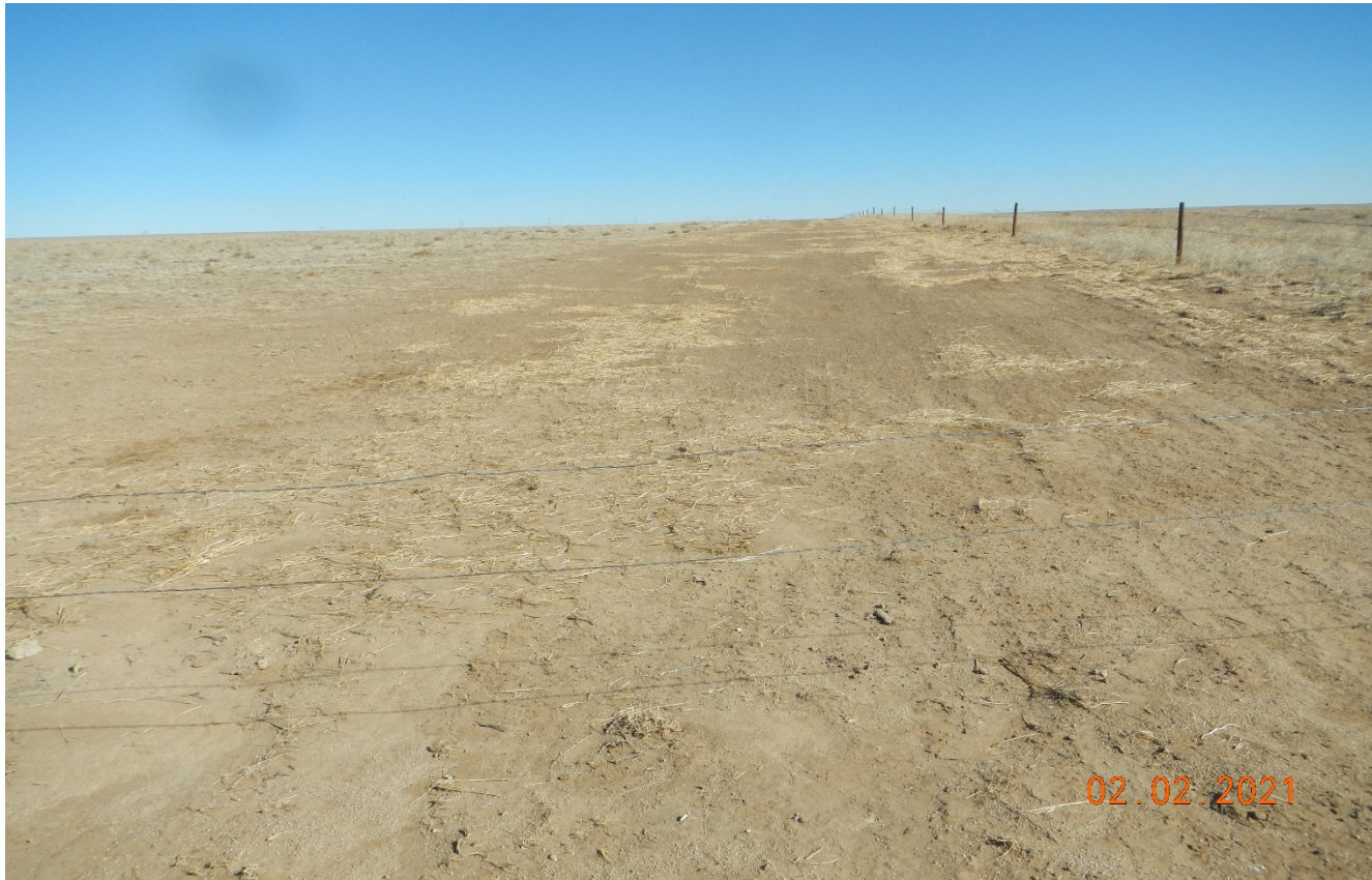
Photo 1. Facing east at the beginning of the access road. The road has recently been reclaimed. Straw mulch was applied to the soil however, much of the straw has blown away in this area of the road.
