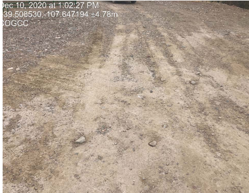
Previous inspection photo of lack of stabilization
