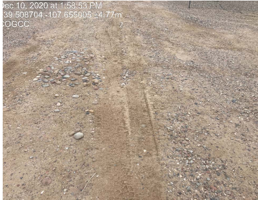
Previous inspection photo of lack of stabilization
