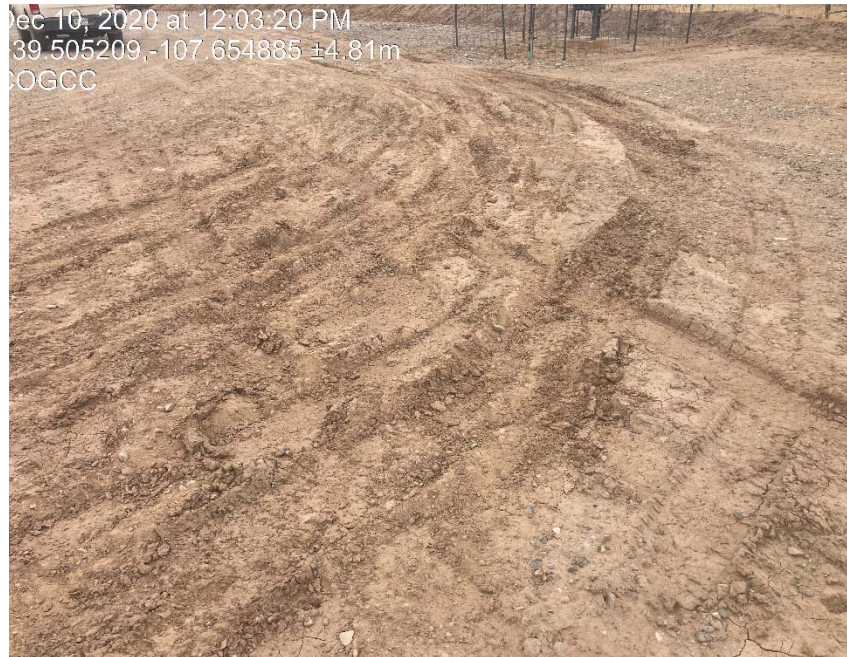
Previous inspection photo of lack of stabilization
