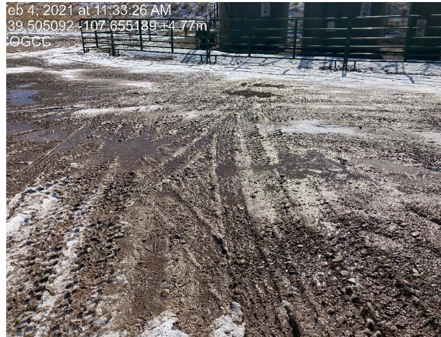
Follow up inspection photo shows that nothing has been done about the lack of stabilization on the pad
