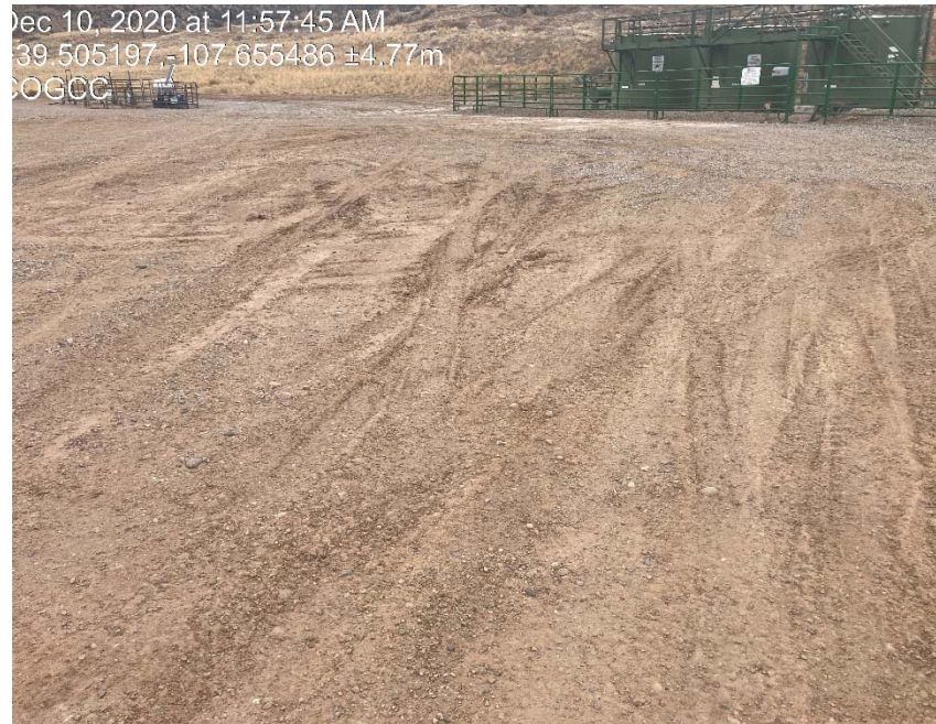
Previous inspection photo of lack of stabilization
