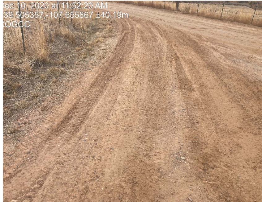
Previous inspection photo of lack of stabilization
