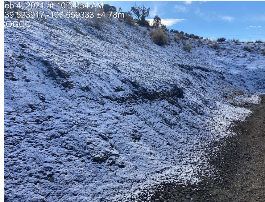
Follow up inspection photo shows that nothing has been done about the lack of stabilization on the cut slope
