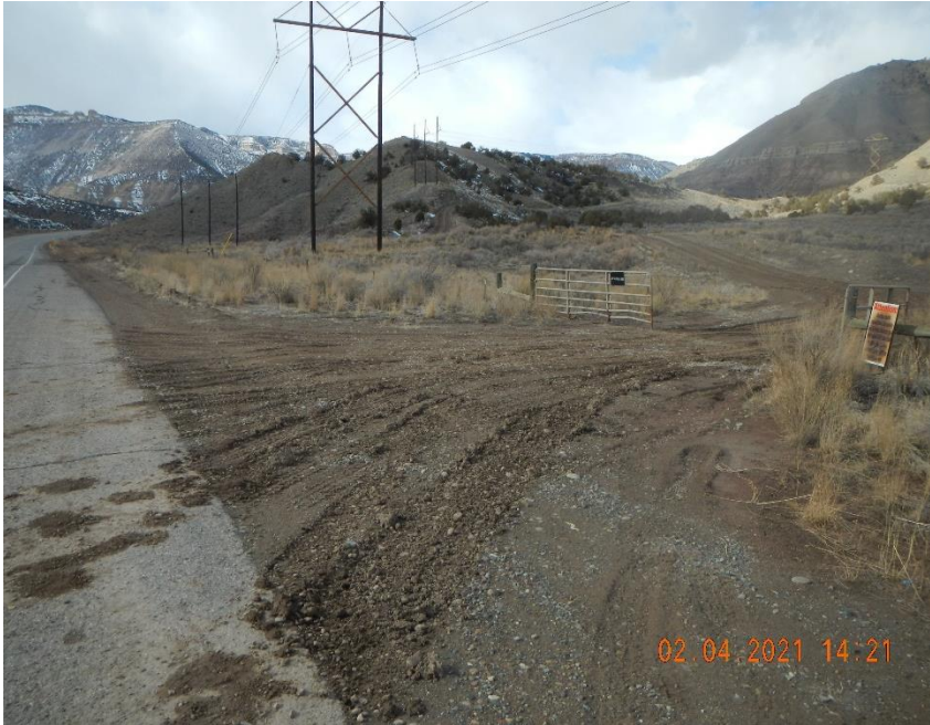
No evidence of tracking control BMP's. Mud tracked on to CR 215.
