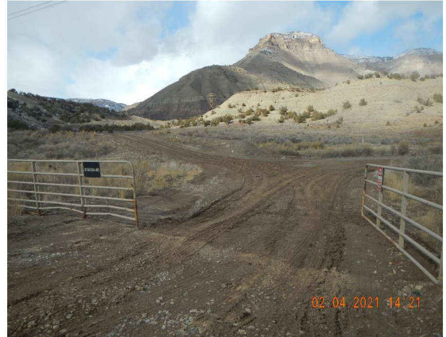
No evidence of tracking control BMP's.
