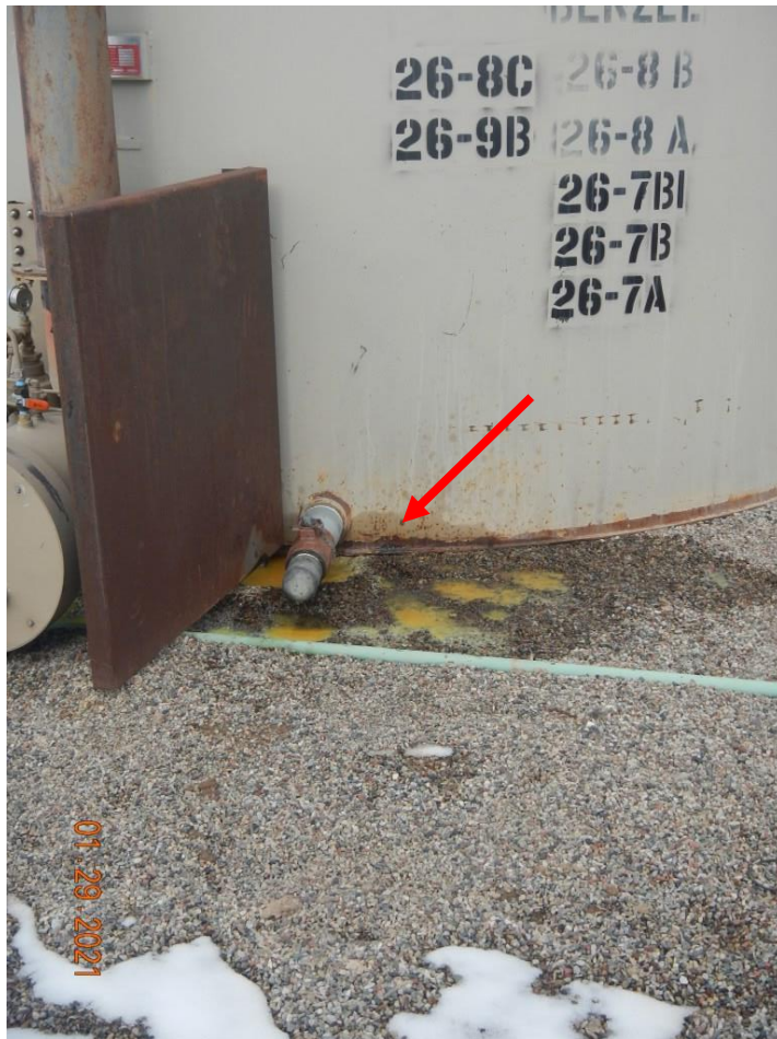
Photo#2: Leaking at base of tank.
