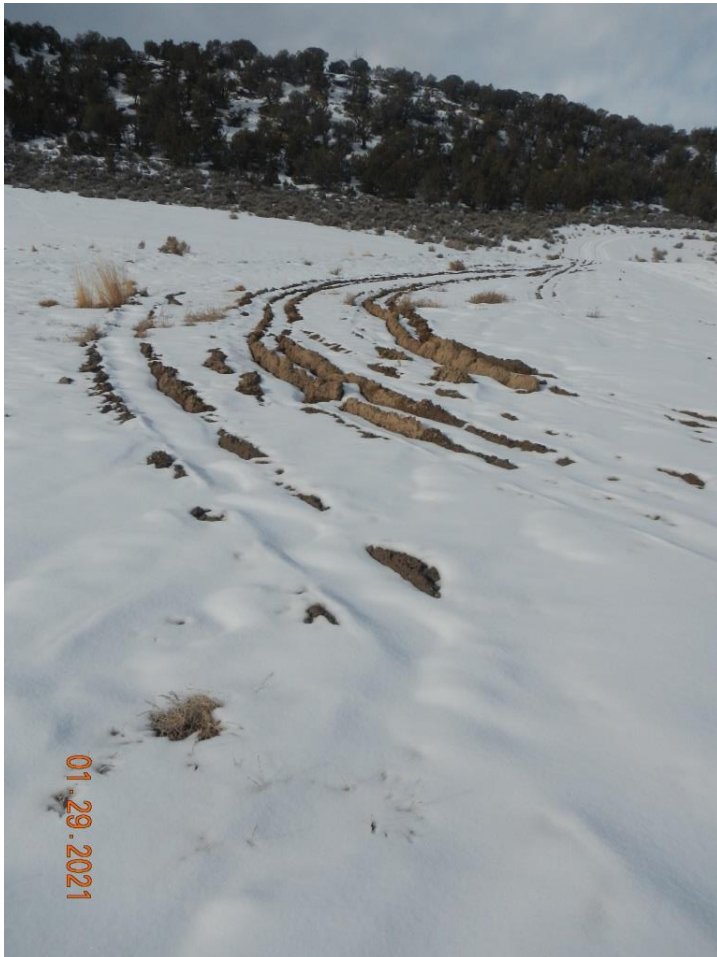
Photo#2: Rutting at Northwest perimeter of Pad.
