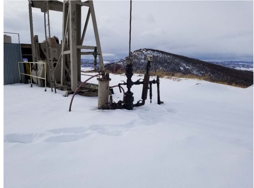
Photo 2. No bradenhead access apparent.
