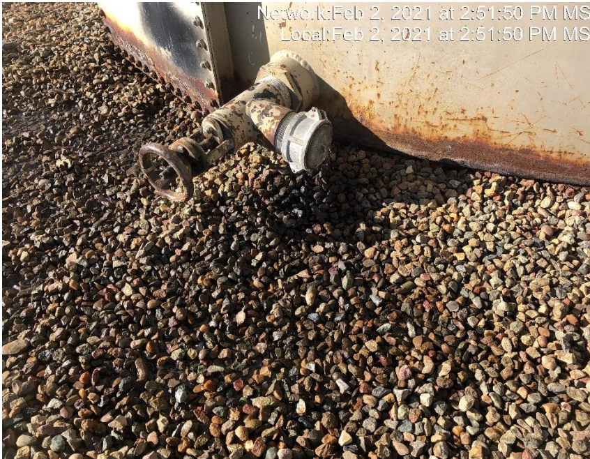
Photo #2797 Stained soils under drain valve.
