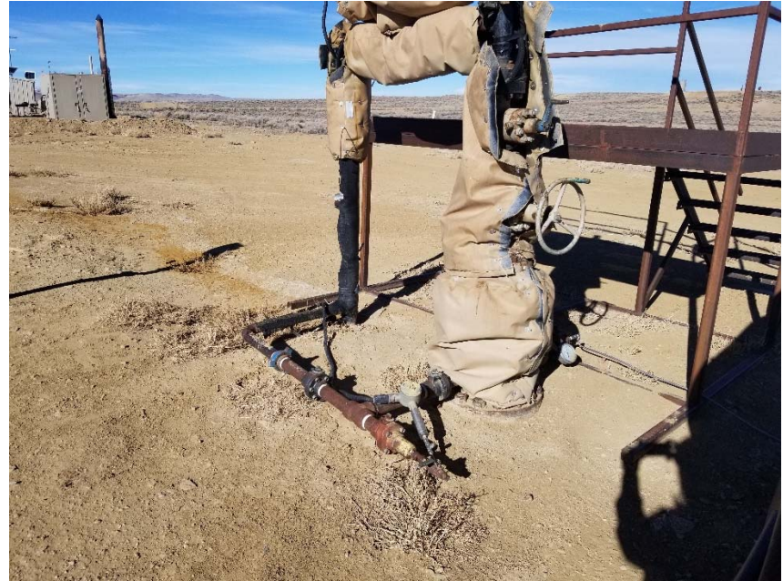
Photo 2. No bradenhead access apparent.
