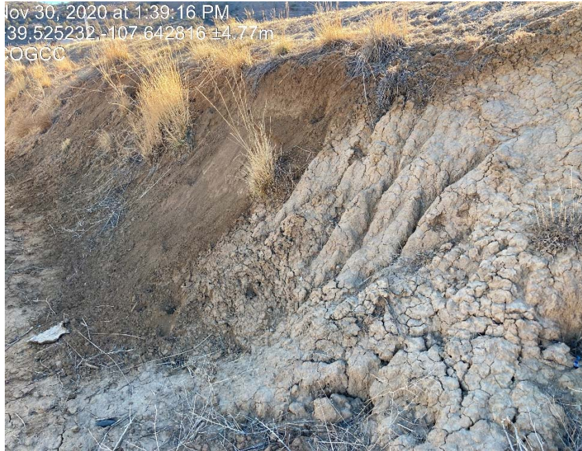
Previous inspection of lack of stabilization
