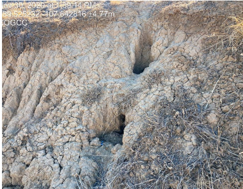
Previous inspection of lack of stabilization
