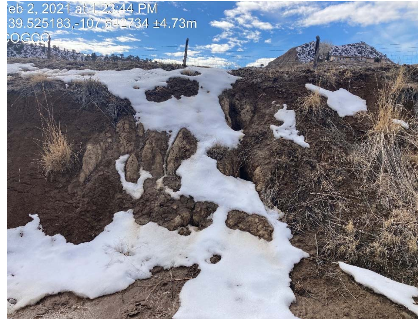
Follow up inspection shows lack of stabilization has not been addressed
