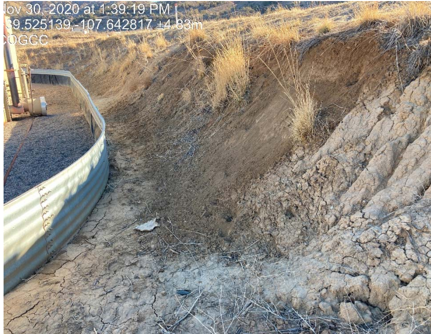
Previous inspection of lack of stabilization
