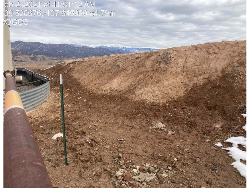
Follow up inspection stabilization has not been addressed
