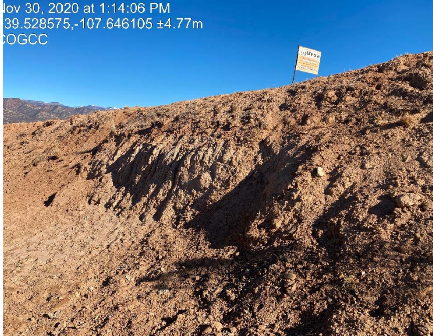
Previous inspection of lack of stabilization
