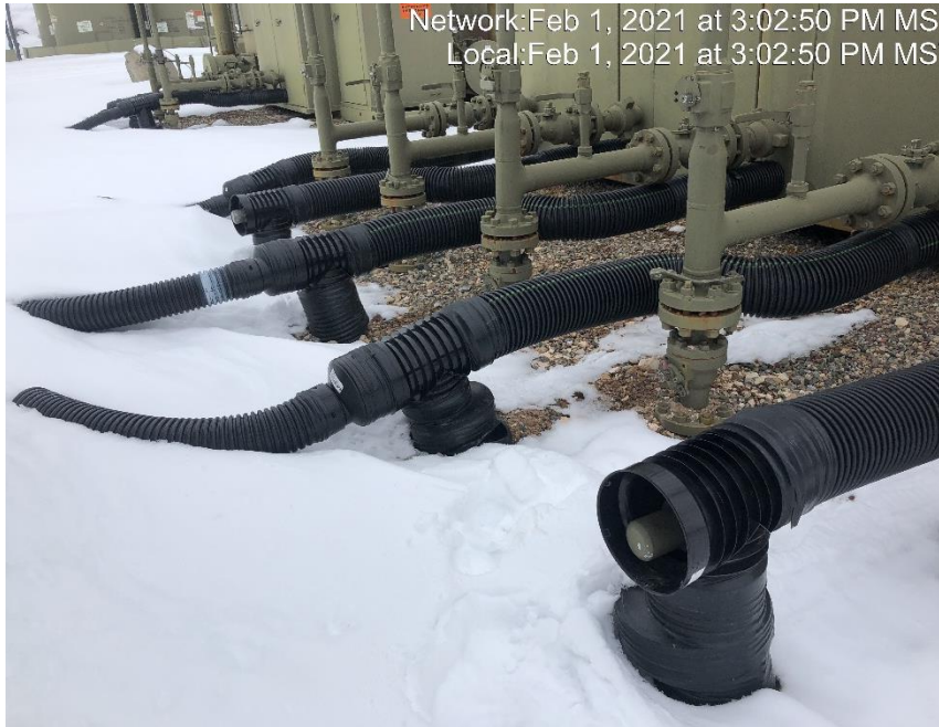
Photo #2787 Flow line exhaust heating insulation open ended and not capped.
