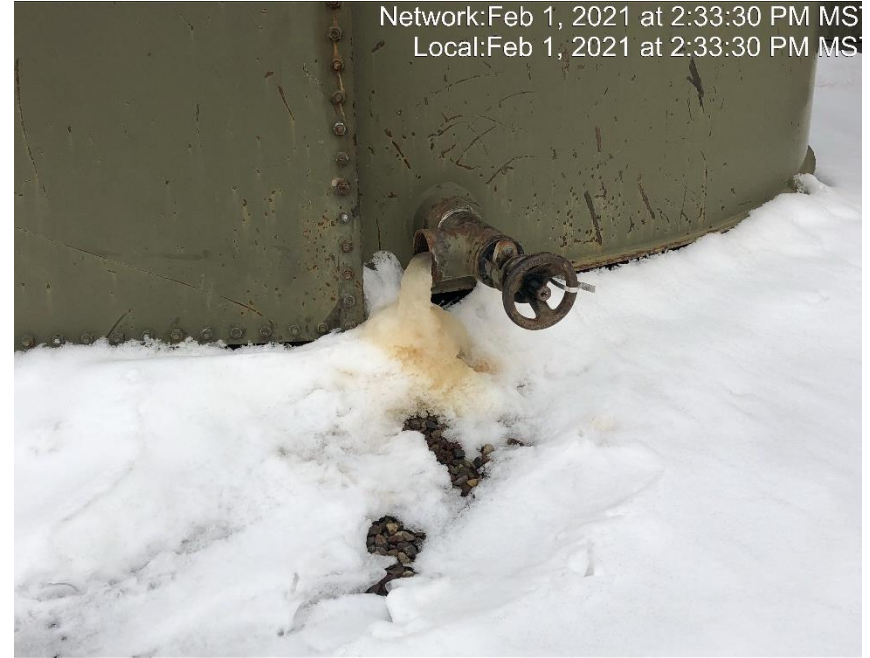
Photo #2780 Drain valve on tank #82965 leaking.
