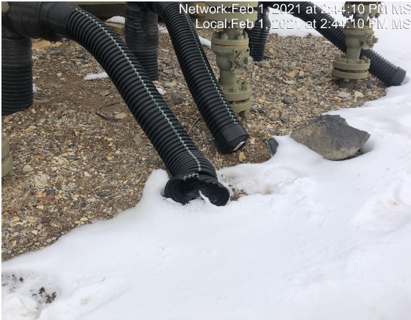
Photo #2783 Flow line exhaust heating insulation open ended and not capped.
