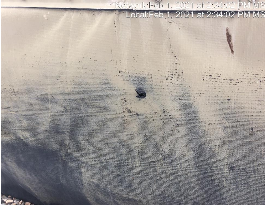
Photo #2781 Hole in tank containment.
