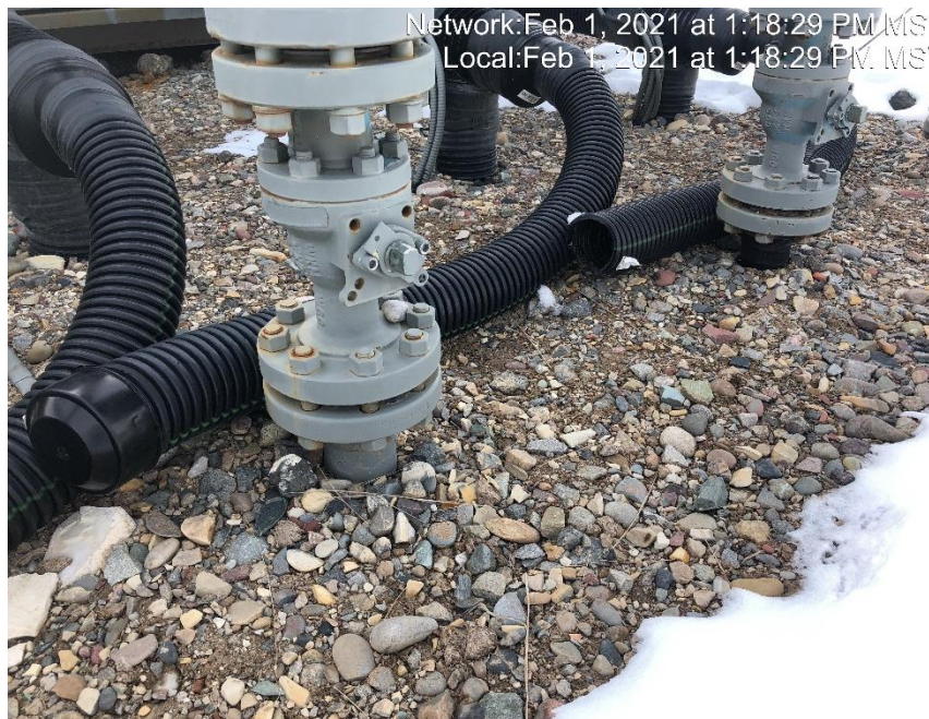
Photo #2770 Multiple places with flow line exhaust heating insulation open ended and not capped.
