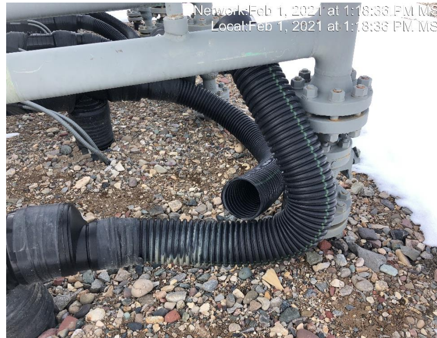
Photo #2771 Multiple places with flow line exhaust heating insulation open ended and not capped.
