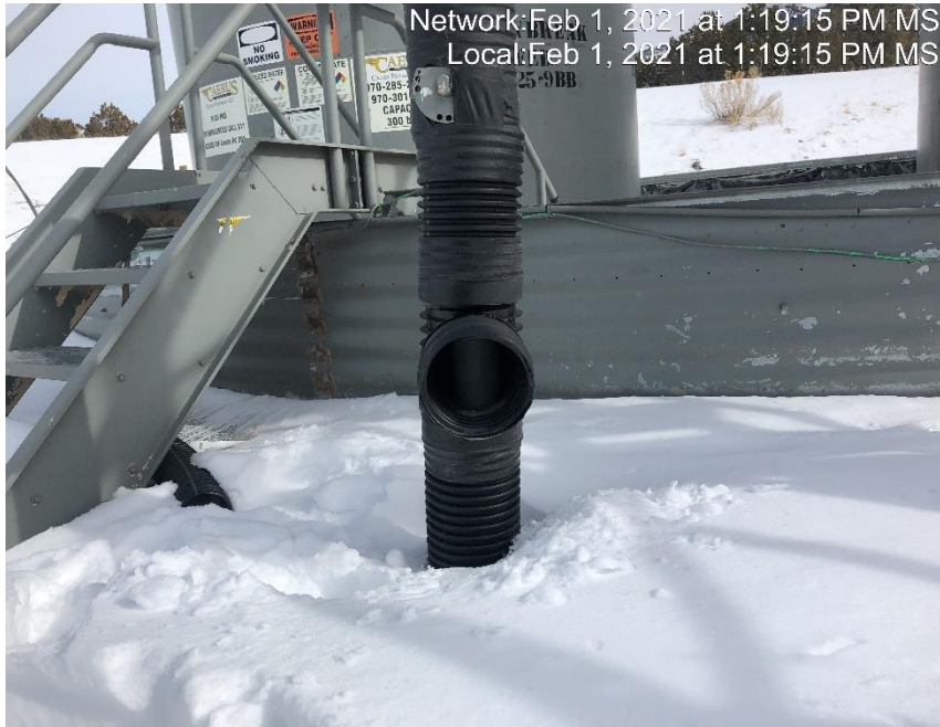
Photo #2772 Multiple places with flow line exhaust heating insulation open ended and not capped.
