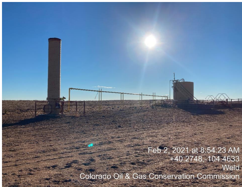
Photo #2 Tank Battery & ECD
