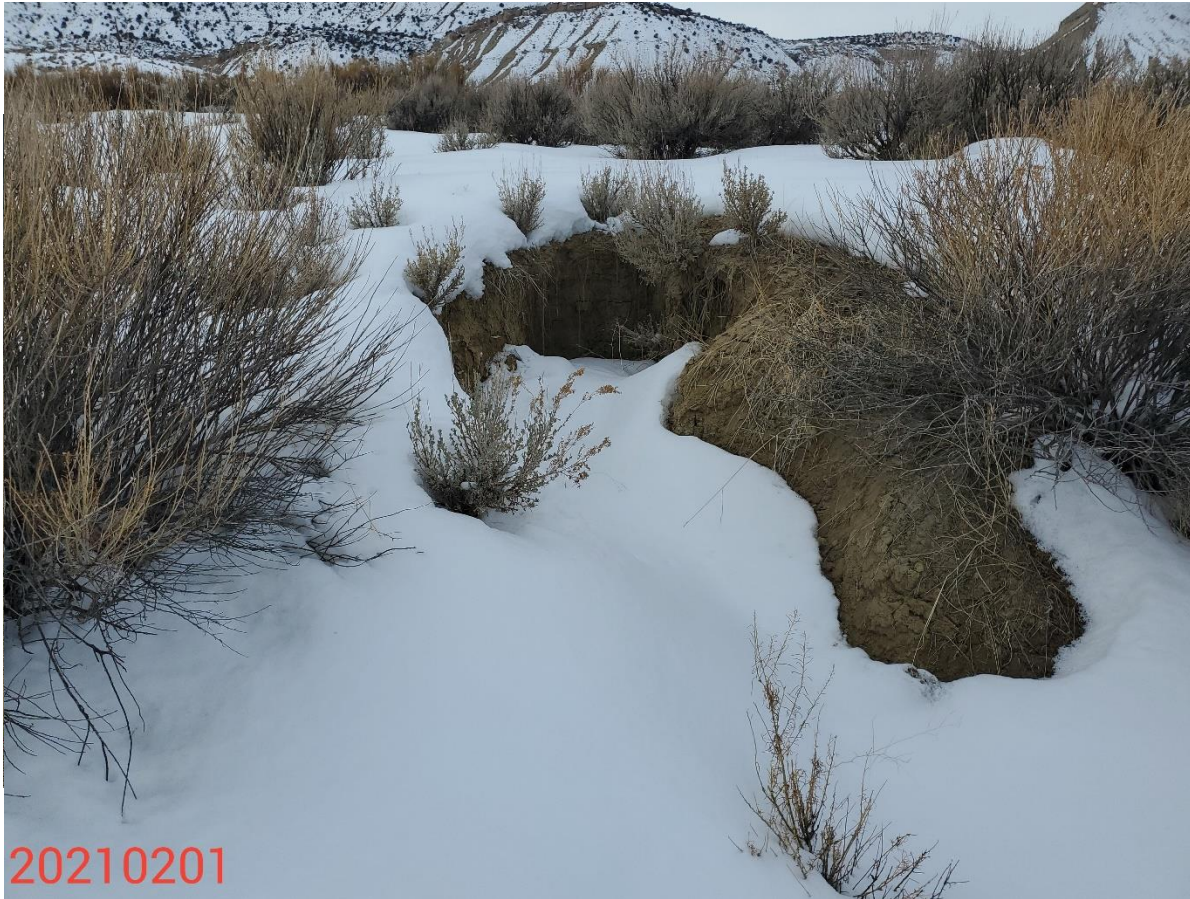
Photo 8: Continued from photo 7. Photo shows gully erosion/head cut.
