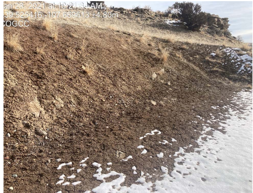
Current inspection photo of lack of stabilization
