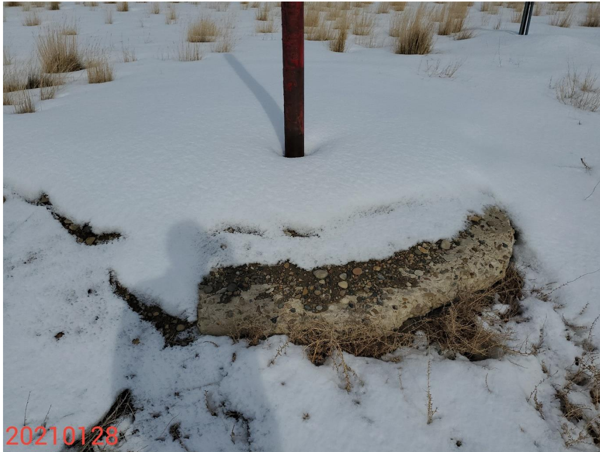
Photo 3: Photo shows concrete base remaining at well. .
