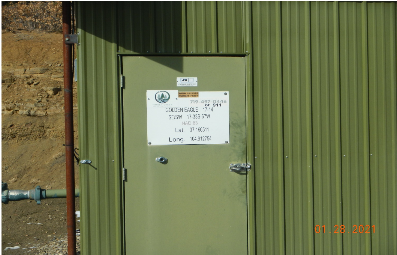
Photo 3. Well sign is posted at meter shed. Operator name will need to be updated.
