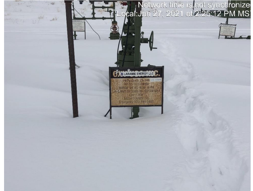
Photo #2738 Multiple wellhead signs weathered and not legible.
