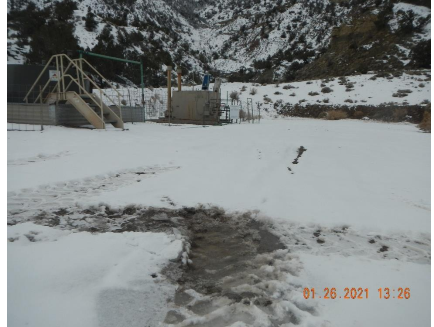
Location shows signs of lack of stabilization BMP's in some areas (rutting is present)
