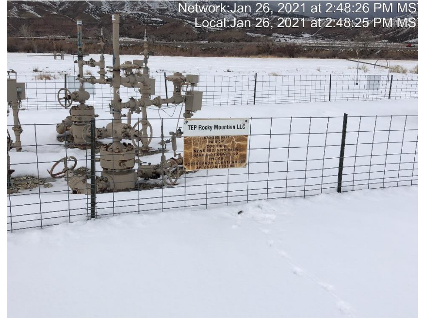
Photo #2726 Multiple wellheads signs weathered and not legible.
