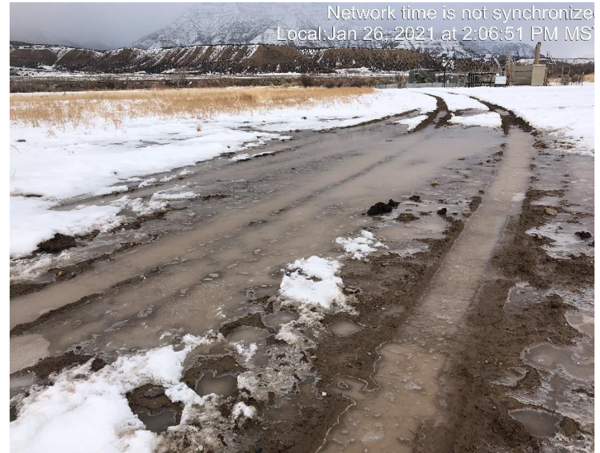
Photo #2721 Ruts present on location due to lack of stabilization.
