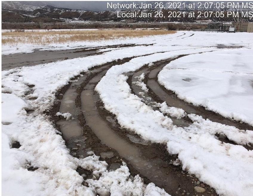
Photo #2722 Ruts present on location due to lack of stabilization.
